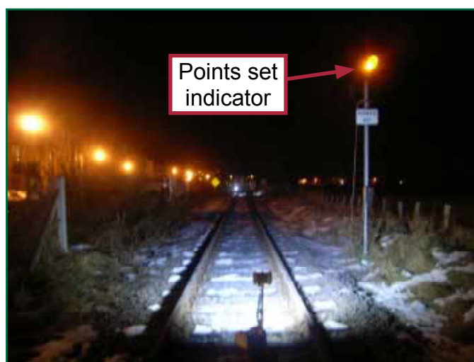
Figure 3: View towards the north showing the illuminated points set indicator
