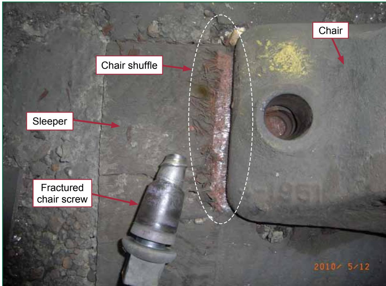
Figure 9: Chair shuffle at derailment site
