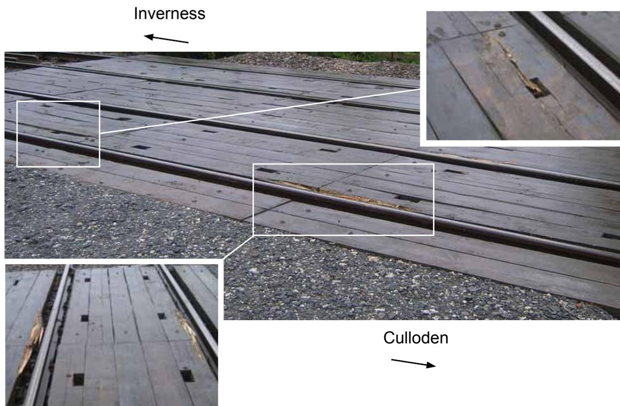
Figure 12: Detailed pictures of damage to Drumrosach RRAP
