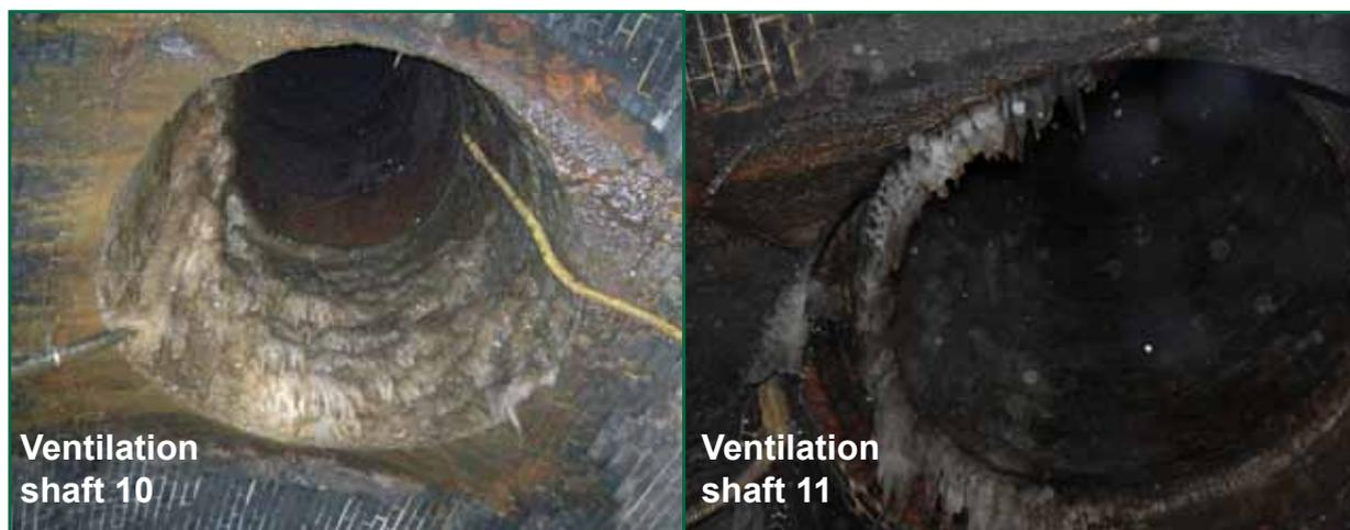
Figure 11: Views looking up at ventilation shafts 10 and 11 showing ice still present in the bottom of the shafts (ventilation shaft 11 photograph courtesy of British Transport Police)
