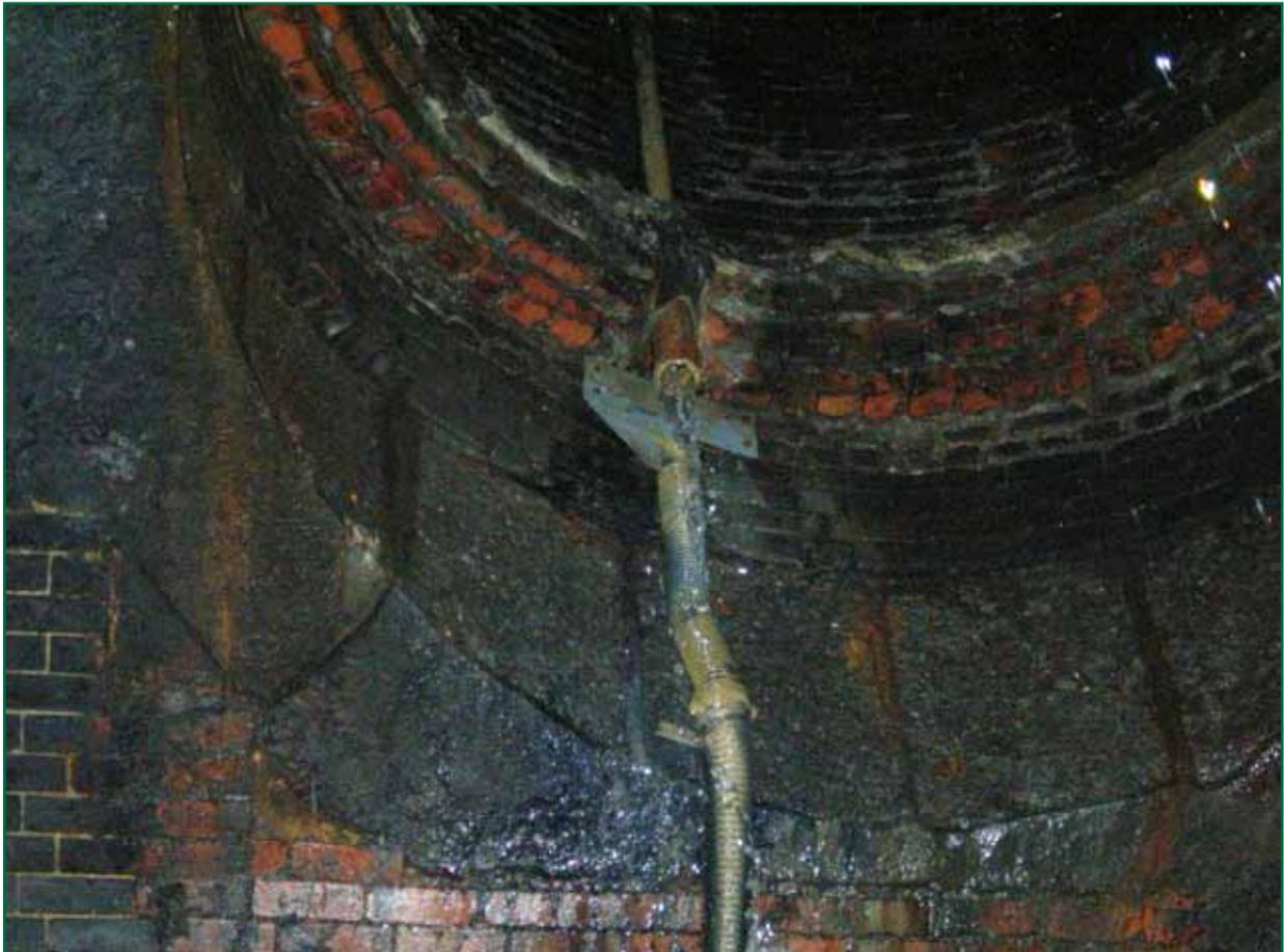
Figure 16: The broken downpipe in ventilation shaft 11
