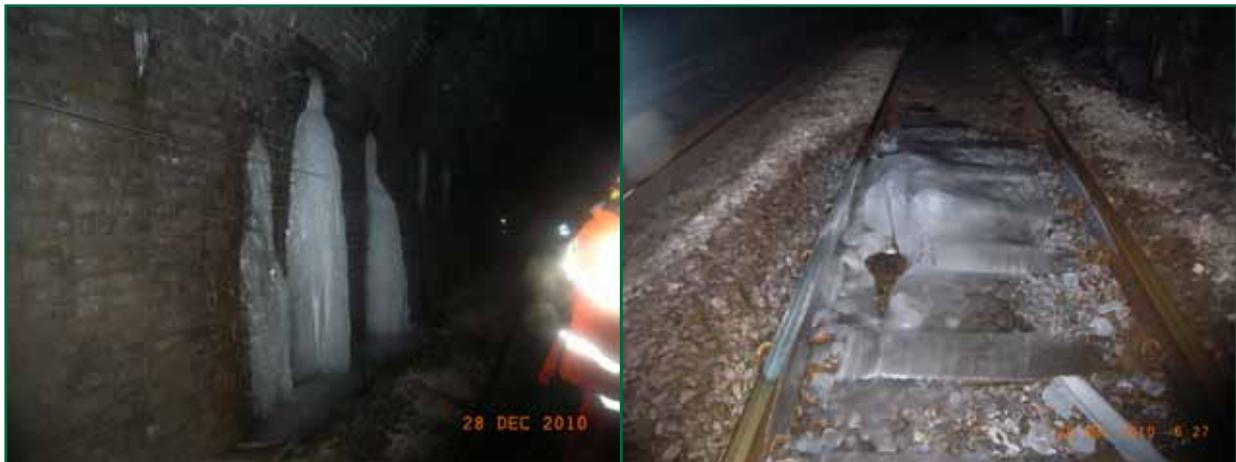
Figure 12: Ice formations found on the track and tunnel wall
