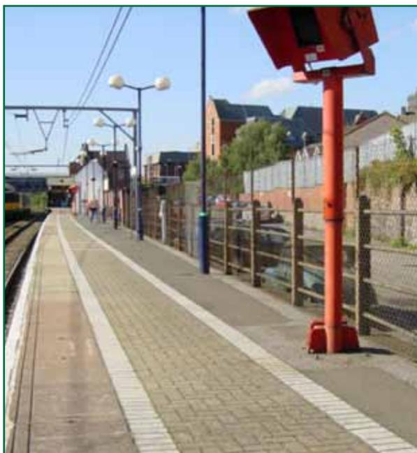
Figure 14: Eight-car monitor position in October 2001. The head of the DOO monitor is rotated to the left and not at an angle to the platform edge (photograph courtesy of Network Rail)
