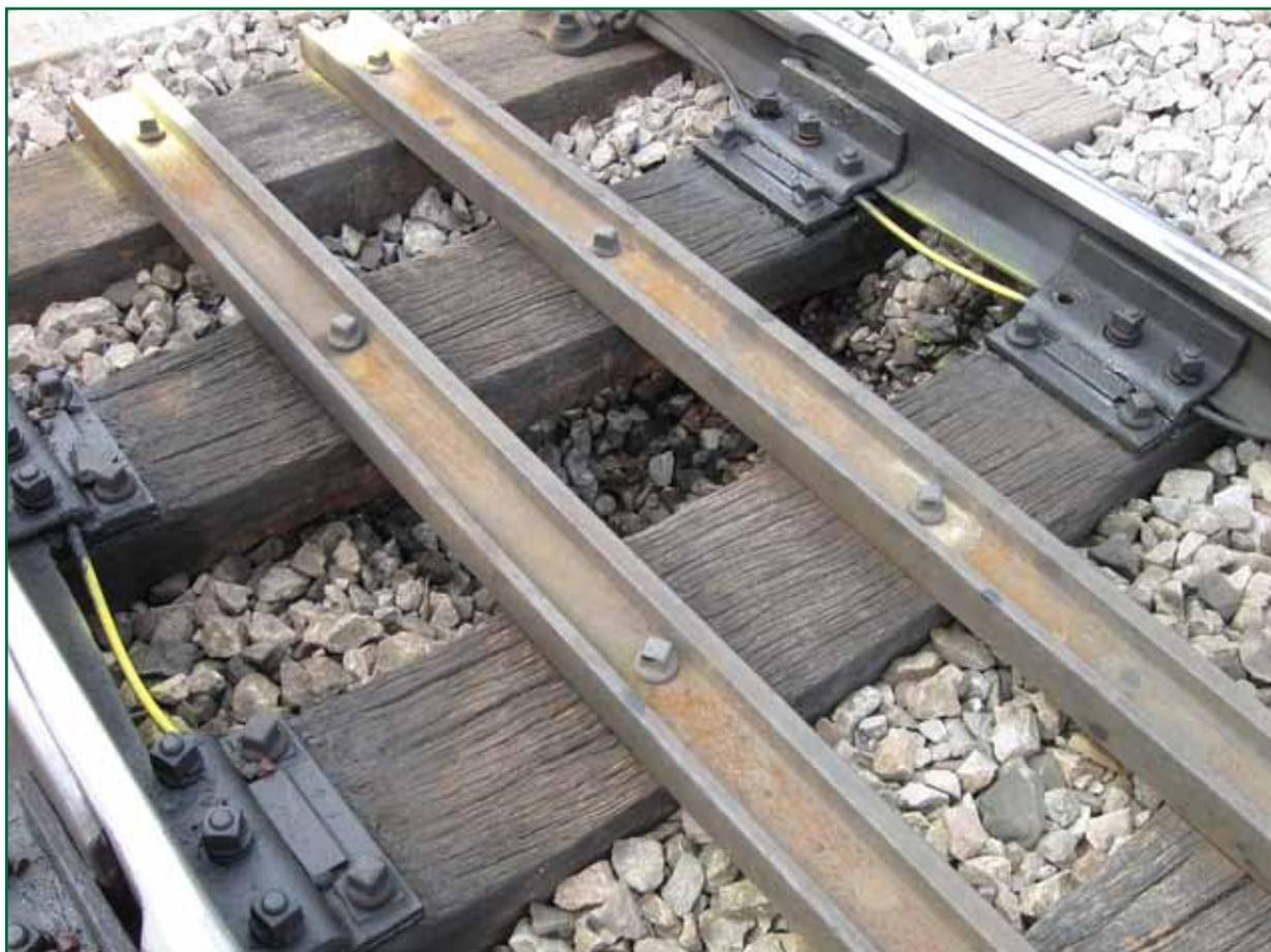
Figure 6: Ballast loss beneath sleepers at adjustment switch (photograph courtesy of Network Rail)
