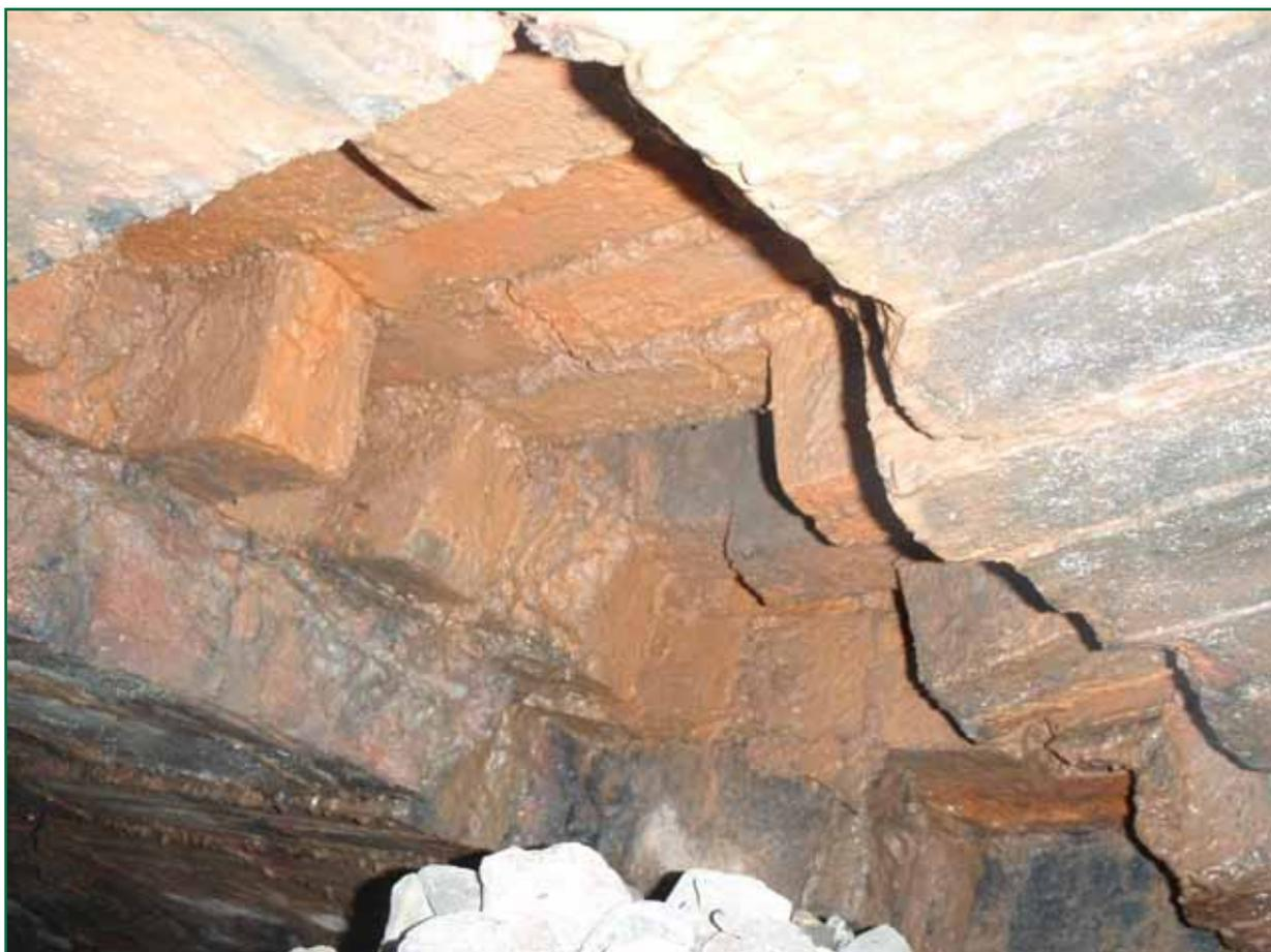
Figure 8: Loss of brickwork at location of failure (photograph courtesy of Amey)
