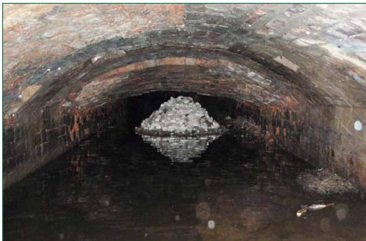
Figure 7: View from within structure showing distortion of arch beneath down main line and ballast lost into watercourse (photograph courtesy of Amey)
