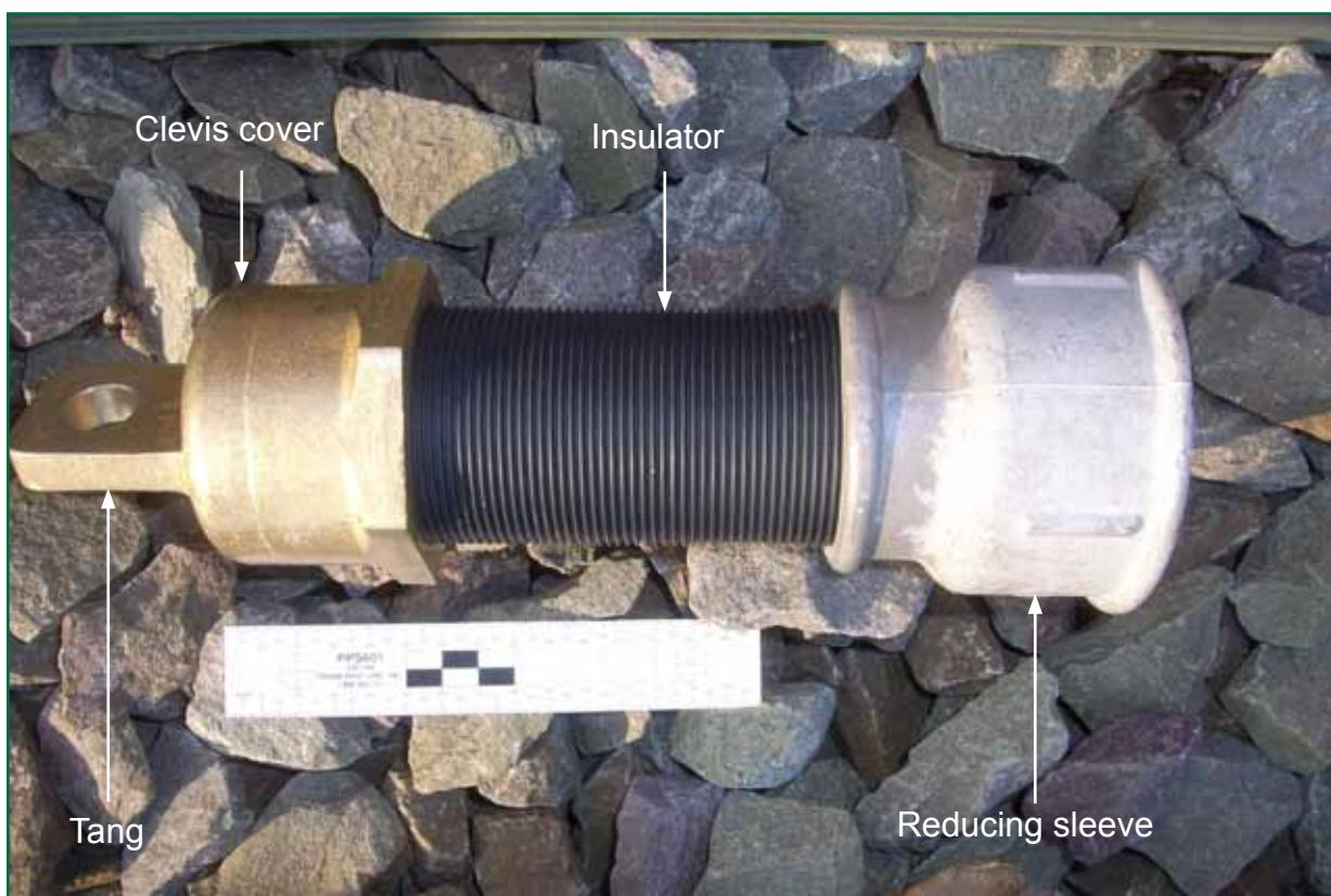
Figure 6: Bracket foot assembly
