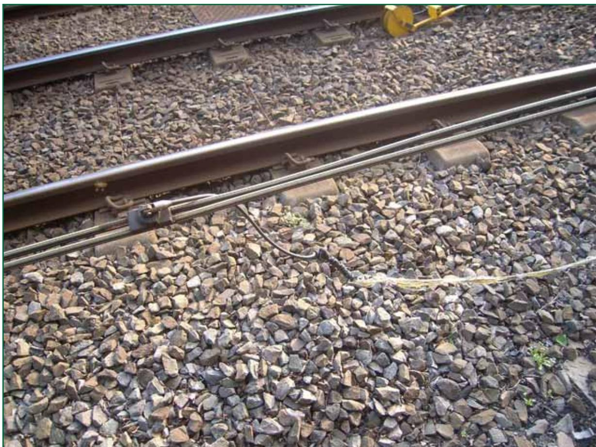
Figure 15: Damage to the delta suspension of the Wolverhampton contact wire
