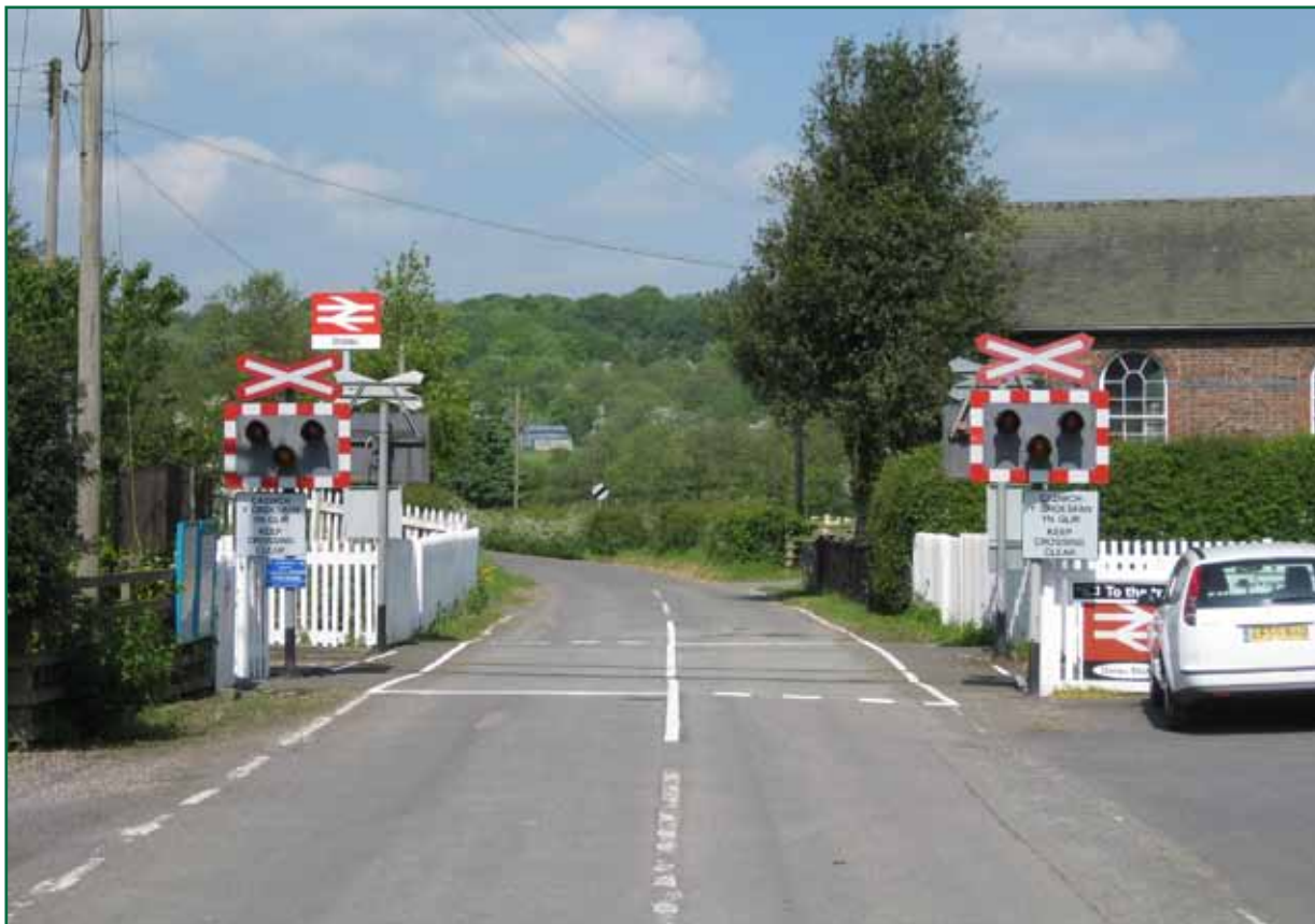
Figure 1: Typical automatic open level crossing (Dolau, Powys)
