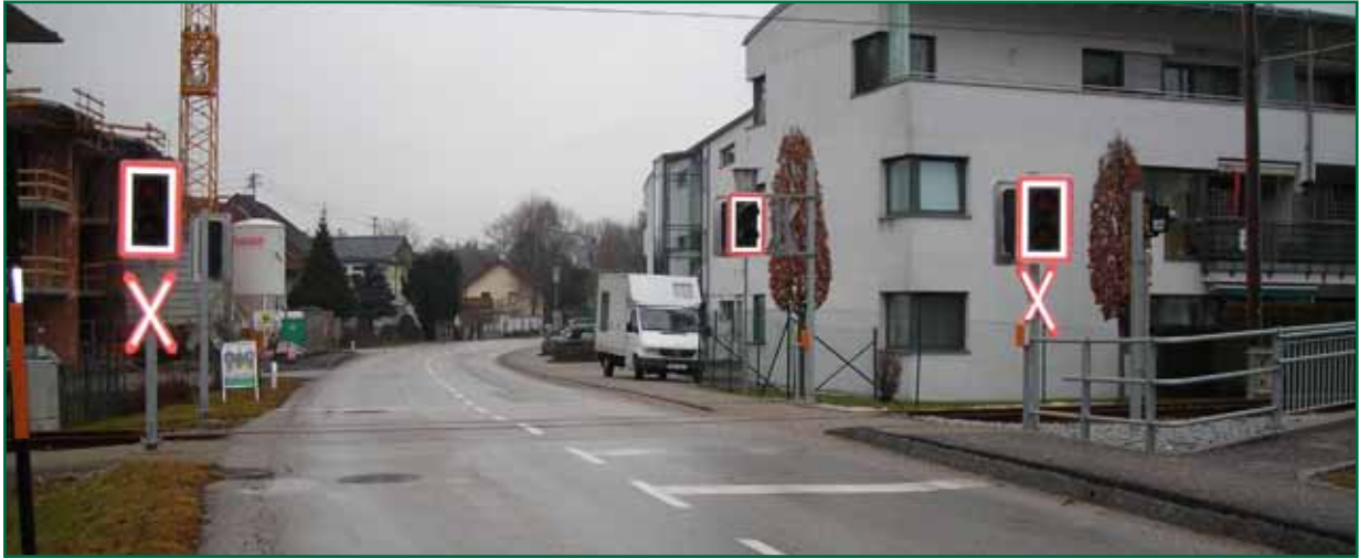
Figure 9: Configuration of road traffic light signals at an Austrian automatic open level crossing (courtesy Austrian Bundesministerium für Verkehr, Innovation und Technologie)
