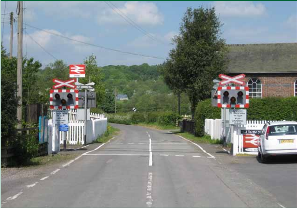
Figure 1: Typical automatic open level crossing (Dolau, Powys)
