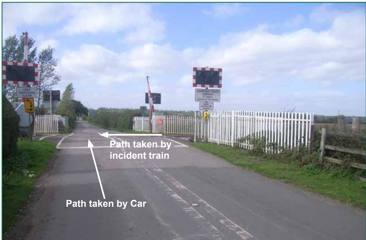
Figure 2: Ufton Automatic Half Barrier crossing looking north west along Ufton Lane
