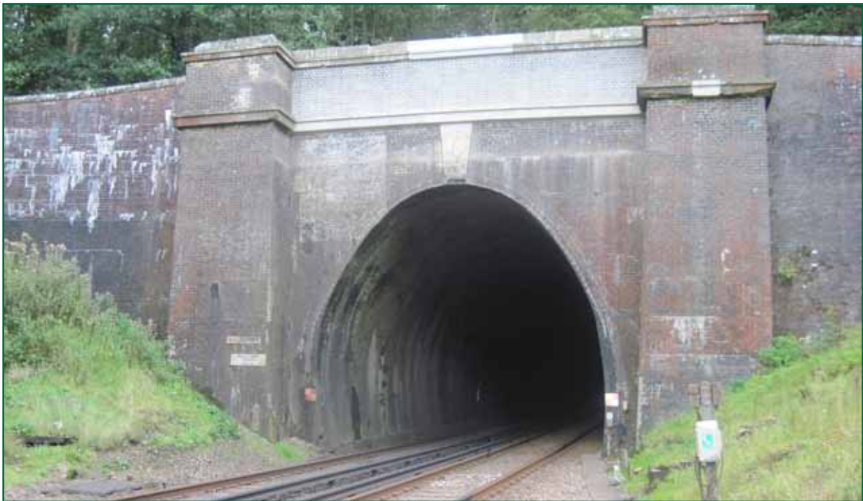
Figure 1: Balcombe tunnel (north portal) (photo courtesy of ORR)
