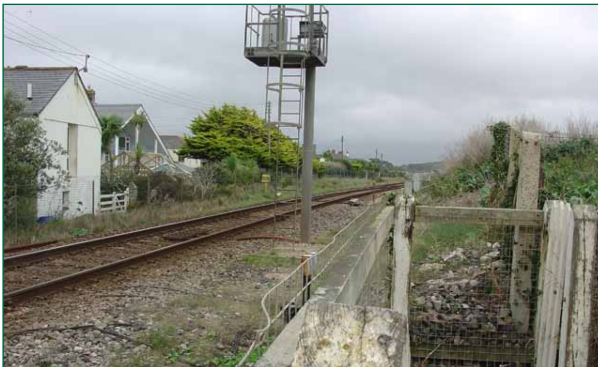
Figure 6: View east from the gate on the south side of the crossing (4.25 metres from the nearer rail)
