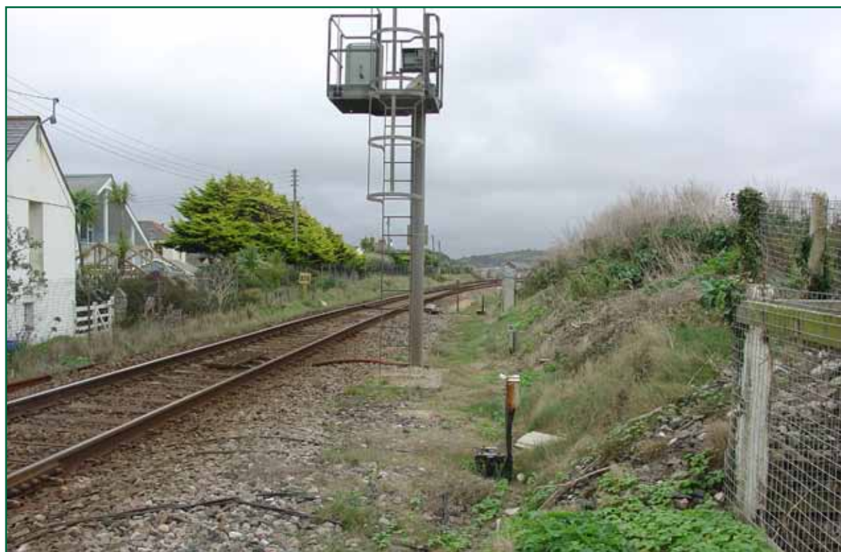
Figure 7: View east from a position alongside the sign on the south side of the crossing (3.40 metres from the nearer rail)
