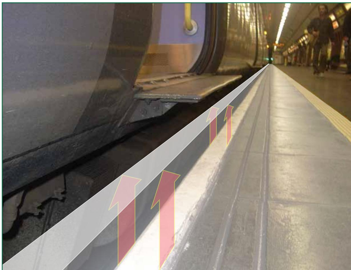
Figure 25: The James Street platform edge gap, shown reduced by raising the platform
