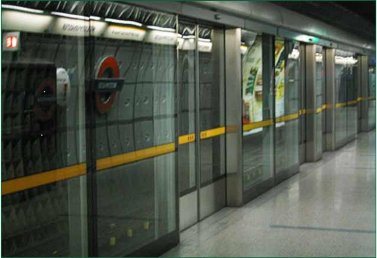
Figure 18: Platform edge doors on London Underground (Courtesy of Transport for London)
