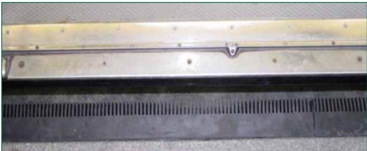
Figure 28: The platform edge after fitting gap filler
