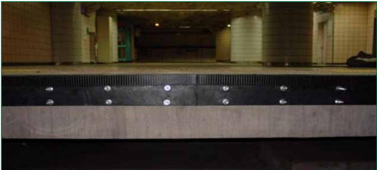
Figure 27: Gap filler bolted to the platform edge
