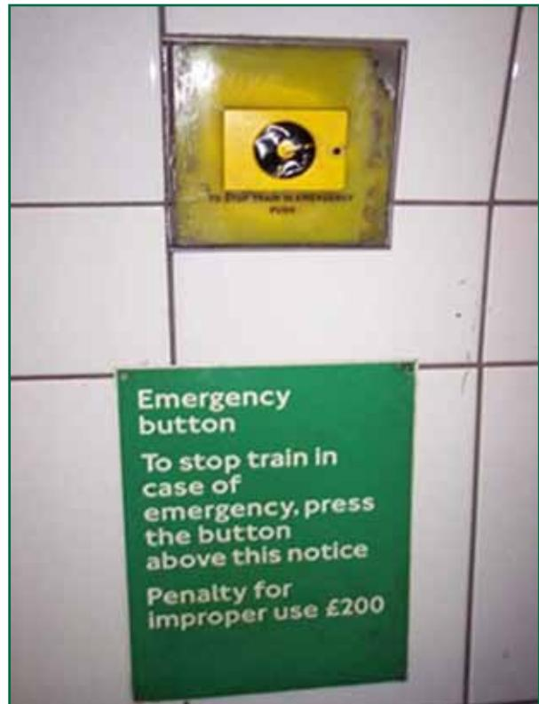
Figure 17: Platform mounted emergency stop button
