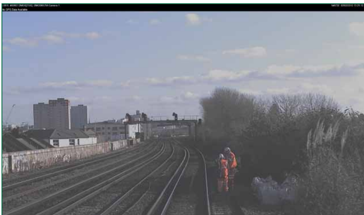
Figure 2: Forward facing CCTV image from train 2N36. The lookout has his back to the approaching train. The COSS is positioned to the right of the lookout. The supervisor is just beyond the COSS and cannot be seen in this image.
