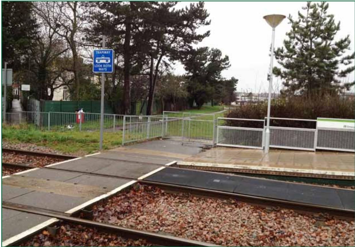
Figure 6: Barriers installed at Arena tram stop
