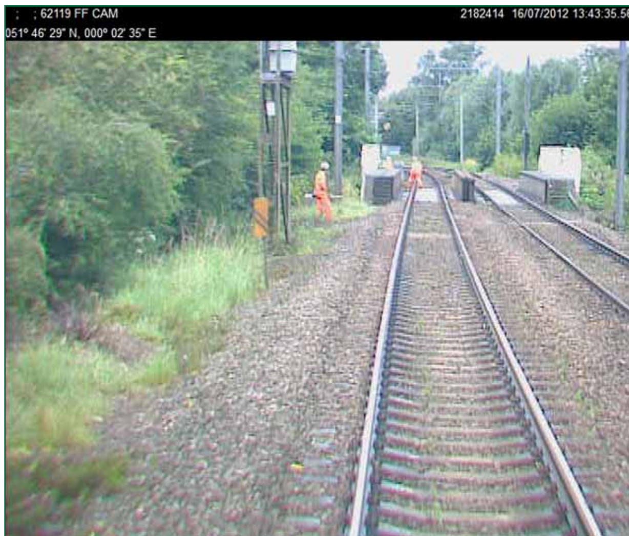
Figure 1: Forward facing CCTV image from train 2H33. The two track workers can be seen on the track and moving towards the south end of the bridge.
