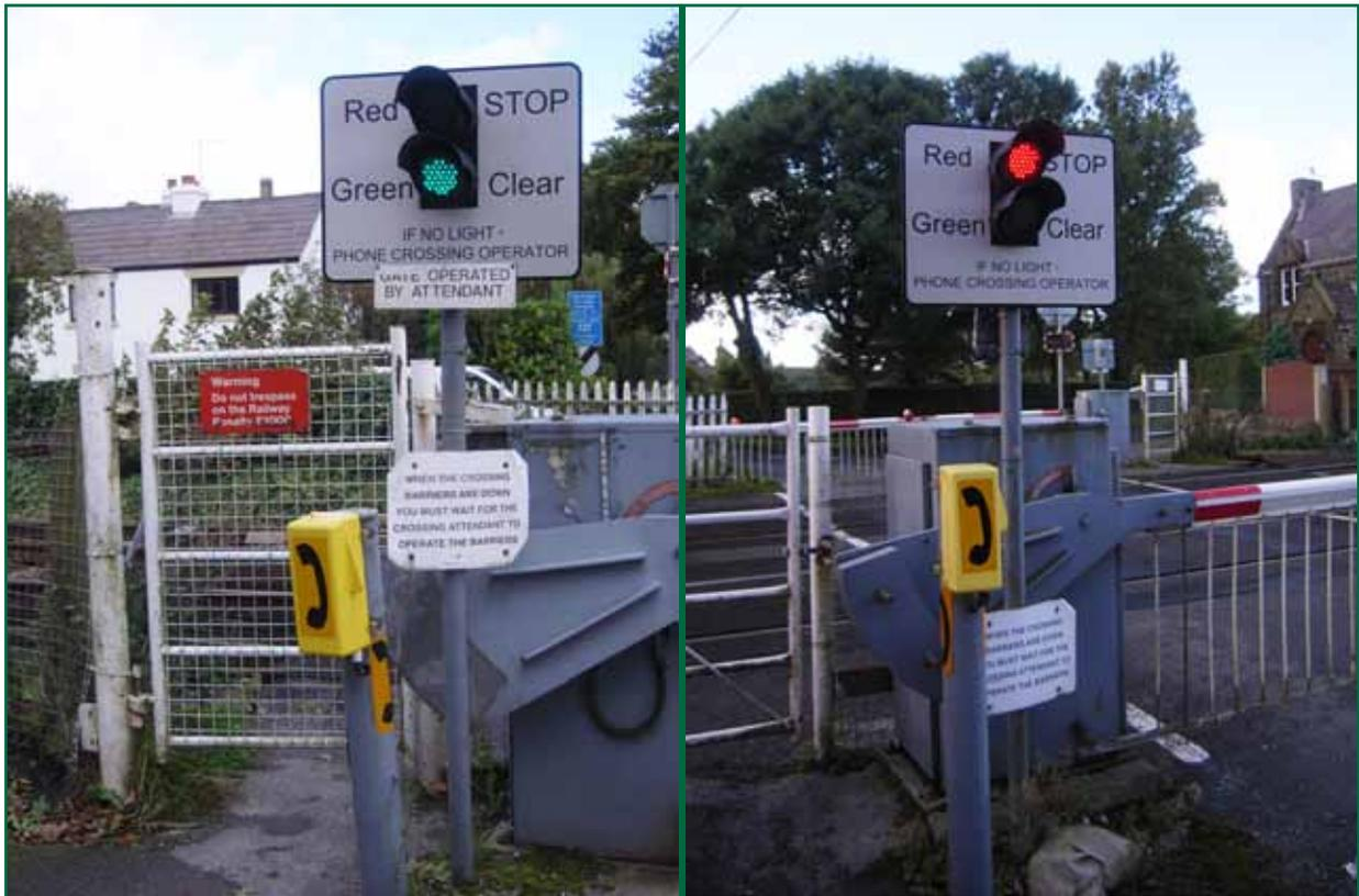
Figure 3: The miniature stop lights at Four Lane Ends crossing
