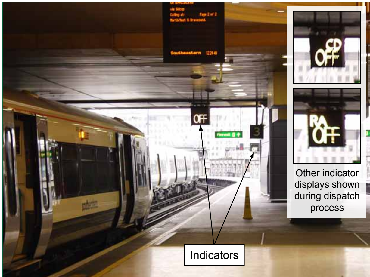
Figure 4: Dispatch indicators on Charing Cross platform 3
