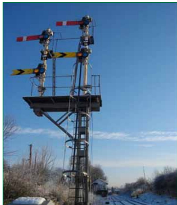
Figure 4: Trees providing a dark background behind the signal structure (left) and the red and yellow light lenses of signal NW36 and the distant signal below (right). Note that the photographs are taken during daylight and not at drivers' eye level.
