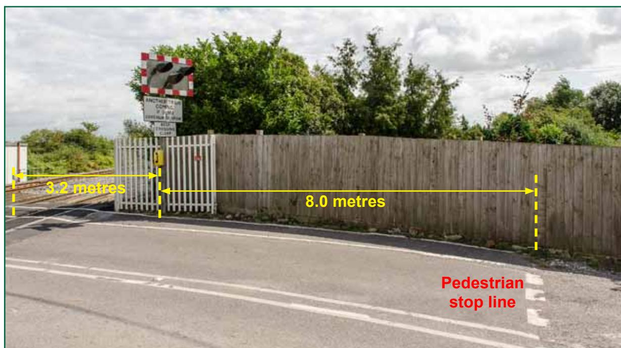
Figure 7: Location of the telephone at Athelney level crossing
