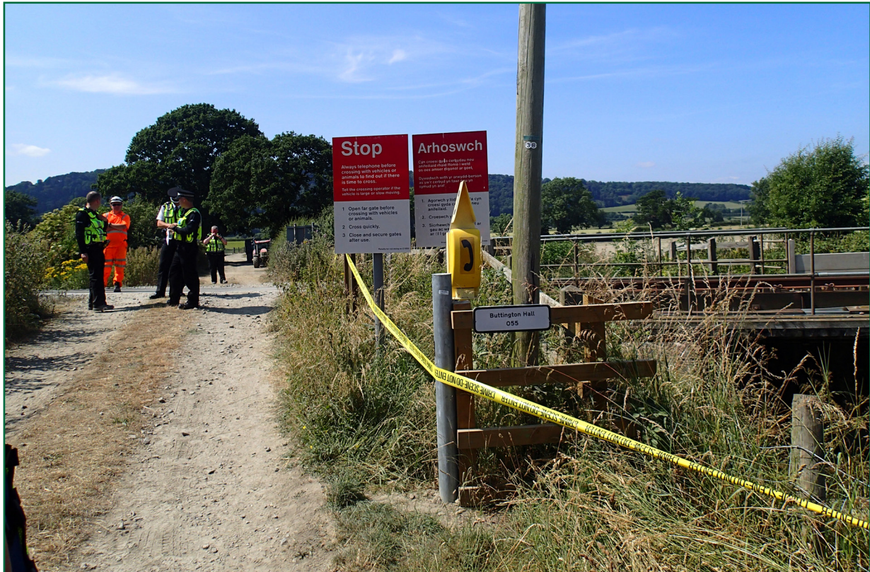
Figure 4: Buttington Hall crossing, looking in the direction that the tractor was travelling, showing the signs and telephone
