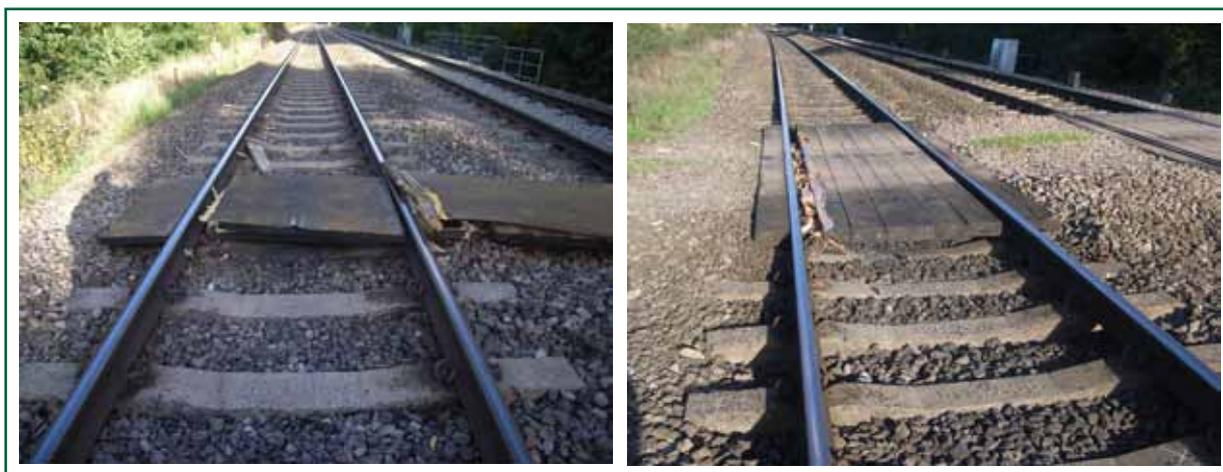
Figure 7: Examples of the damage caused by the derailed wheelset to level crossing surfaces
