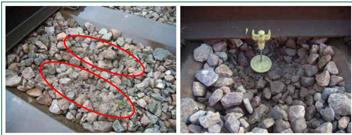
Figure 15: Mud on the surface and contaminated ballast just below the surface
