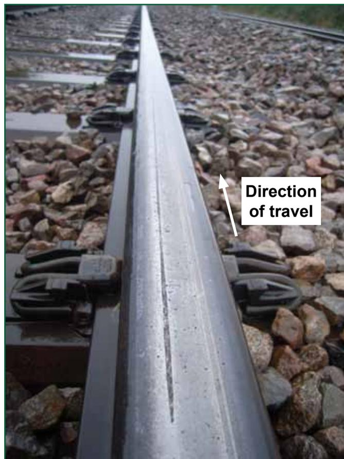
Figure 6: The flange mark on the head of the six foot rail
