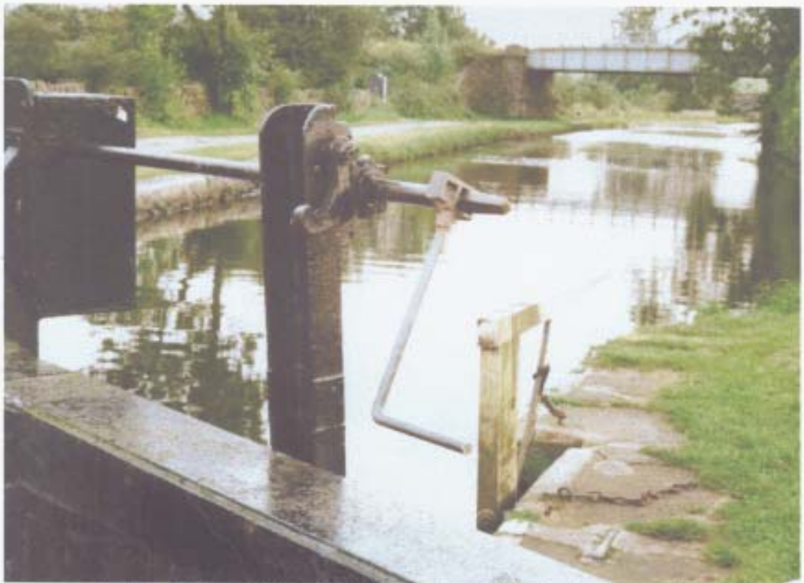
A view of the windlass for the top gate paddle (in foreground) and the wooden lever for the ground paddle (behind).
