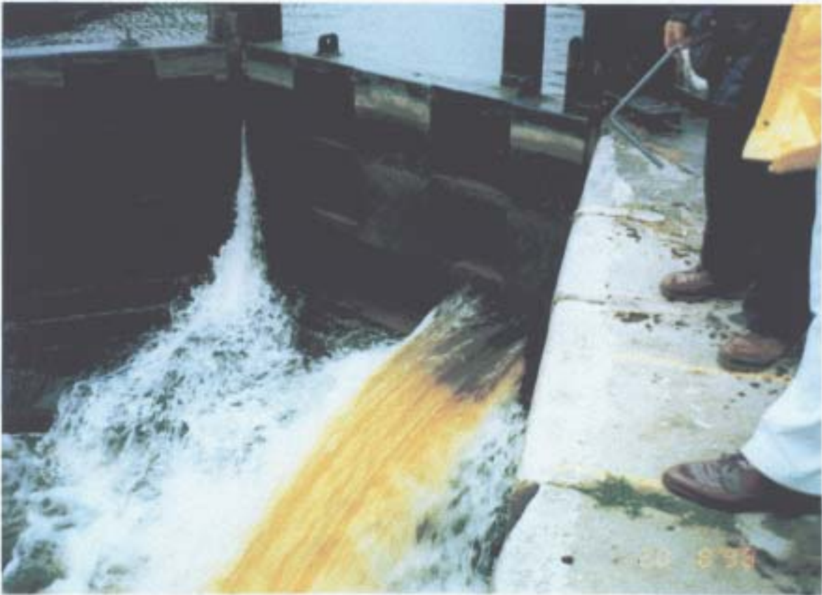
The top paddle gate was opened to show the force of the water entering into the lock. Note the cill beneath and the police yellow chalk marks on the coping stones to the right.
