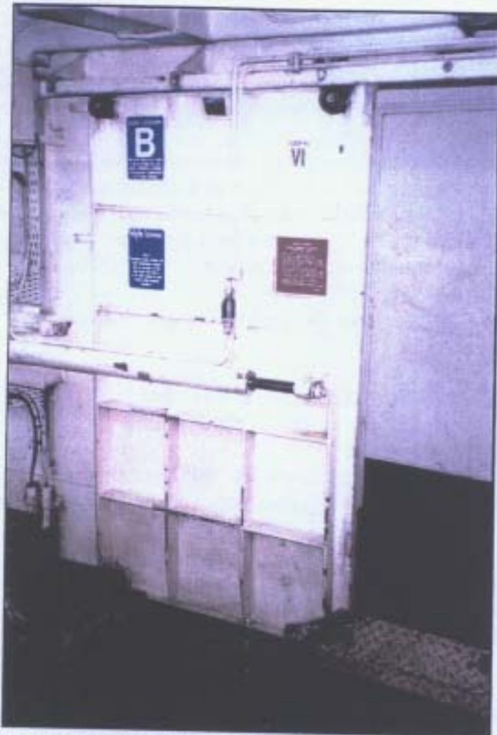
View of raised floorplate when watertight door is partially open.
