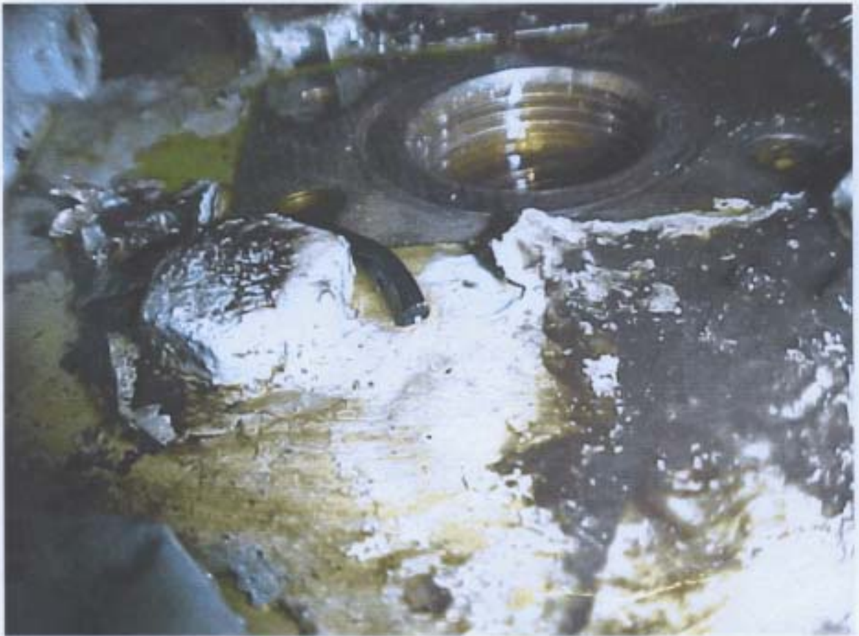
Close up of flange face of O/D box
