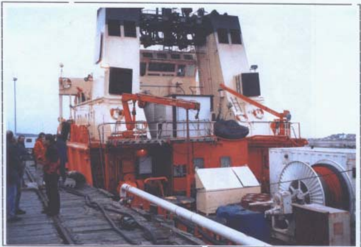
Fig 2 View of accommodation block from aft. Note entrance to the Halon Compartment, port side adjacent to ladder access to forecastle deck.
