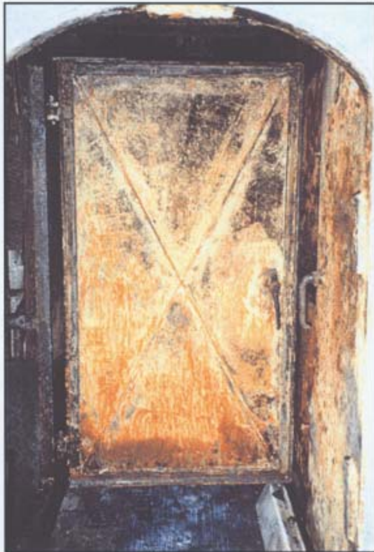
The engine room door open at 90°
