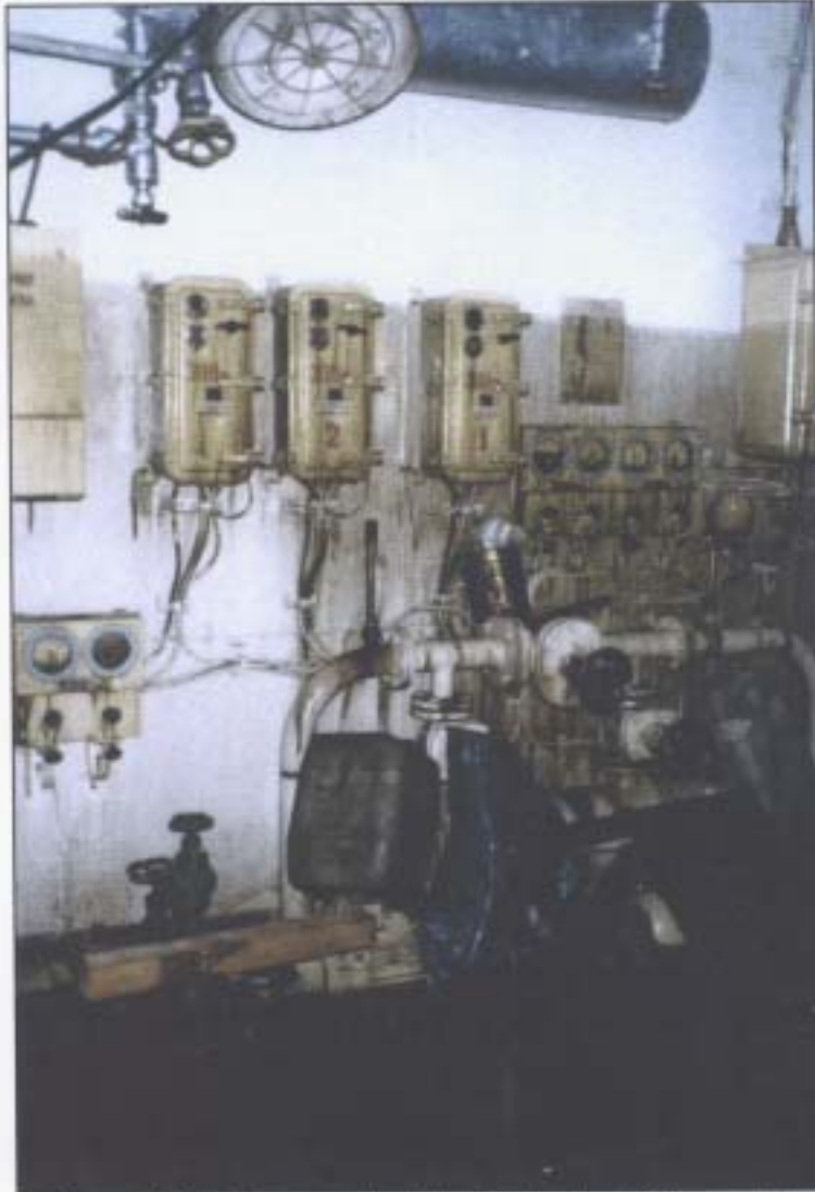
Forward engine room bulkhead showing 'tide mark' of flooding above floor plates
