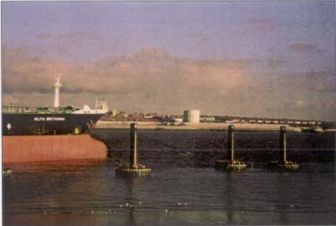
The bow of Alfa Britannia and three of the mooring dolphins at Tranmere oil terminal
