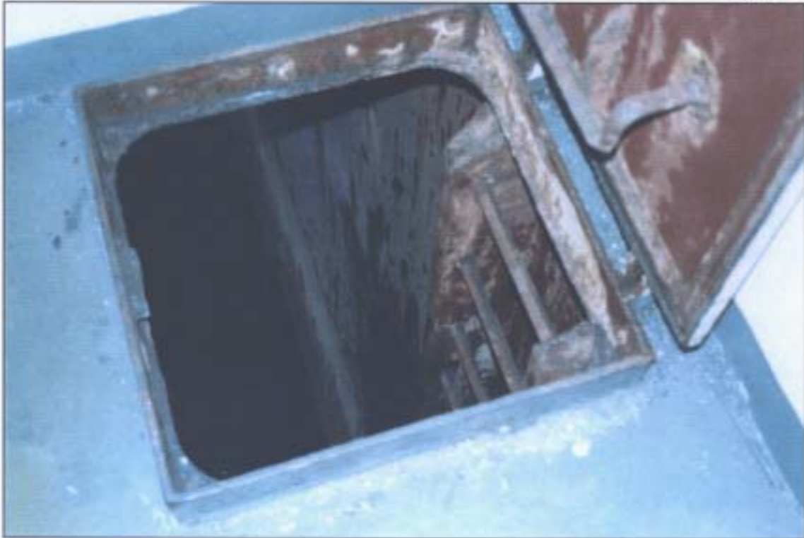
View of entry hatch showing vertical ladder and first platform
