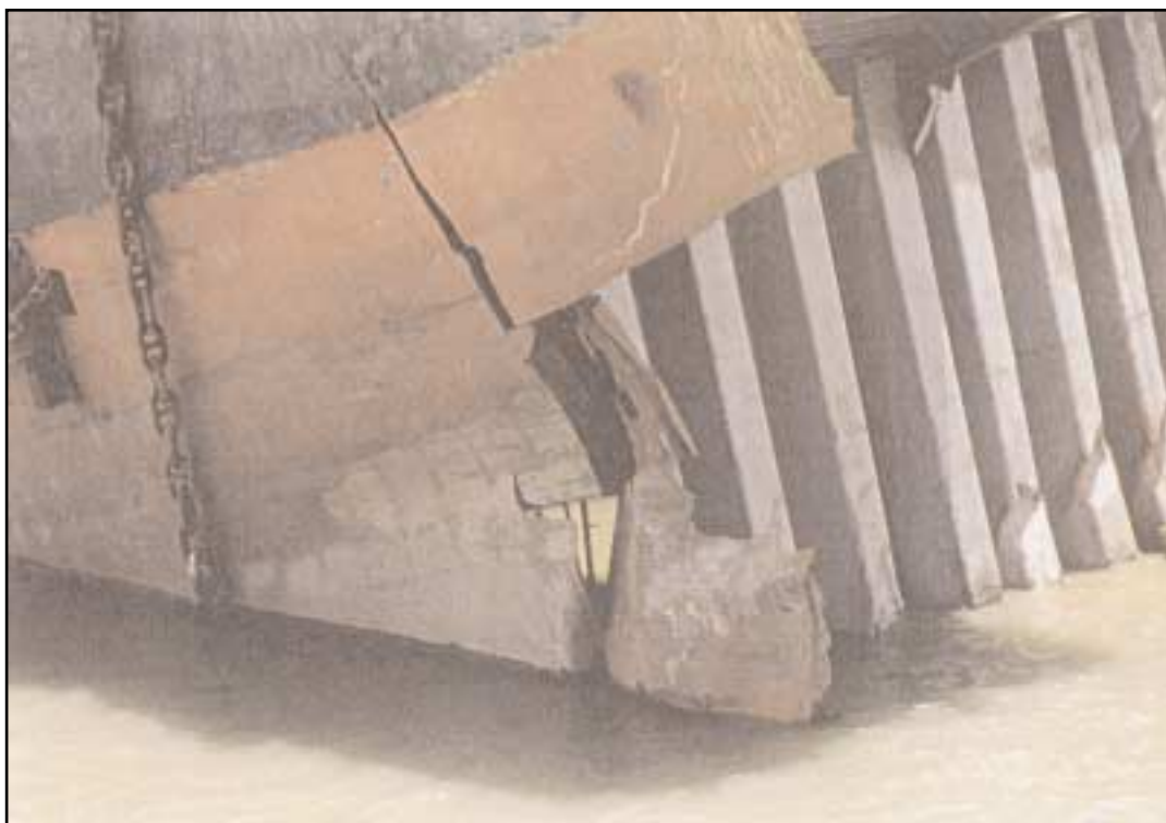
Cut section showing bulb penetration and bulkhead between No 2 and 2a holds
