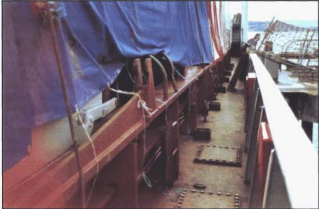
Port side between hatches 2 & 3 showing loose tarpaulin
