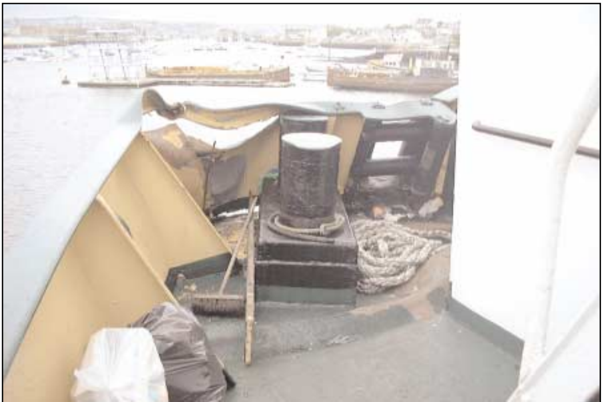
Eastfern - A view of the damage of the starboard side of the poop deck
