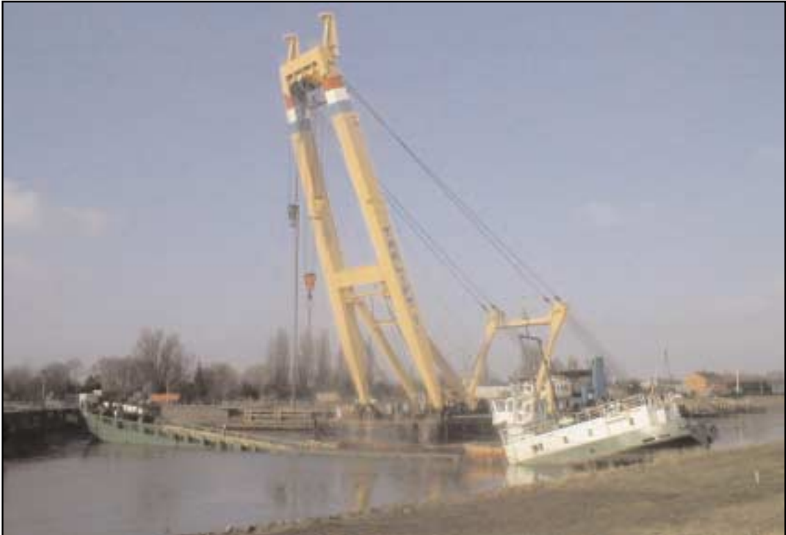
Floating crane moving into position
