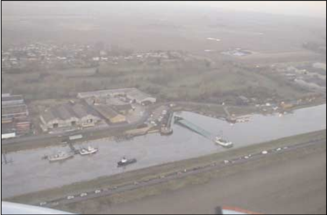
Aerial view from the east (note some pollution)
