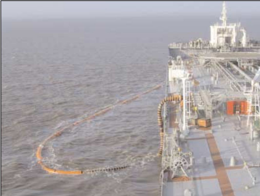
A single floating flexible discharge hose connected between the monobuoy and vessel's discharge manifold
