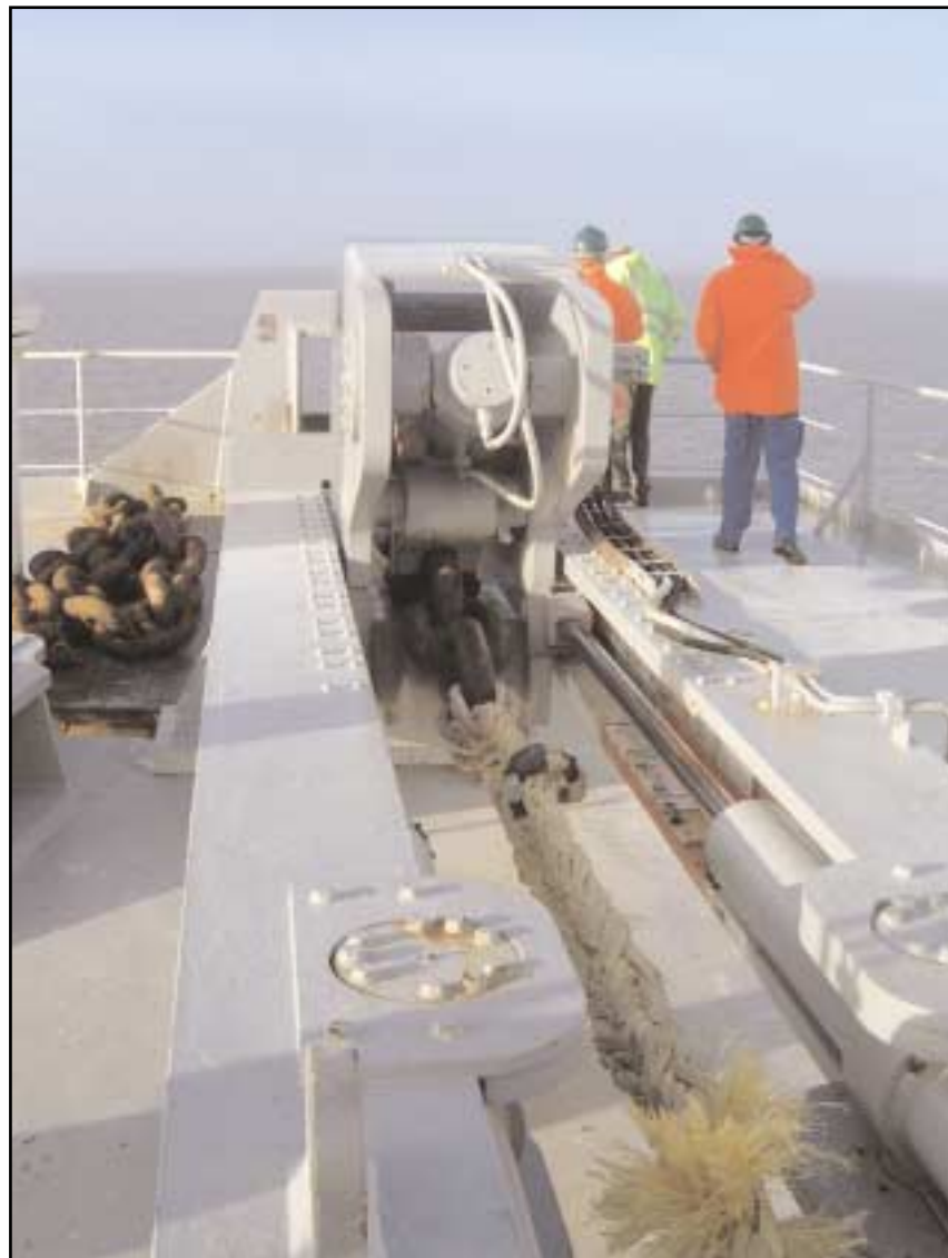
Inboard view of chain stopper showing messenger rope
