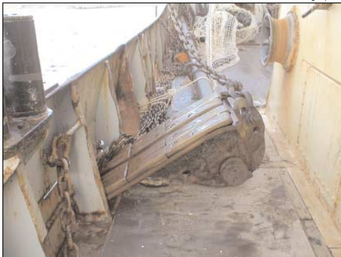
View from aft of the beam shoe having fallen down onto the deck
