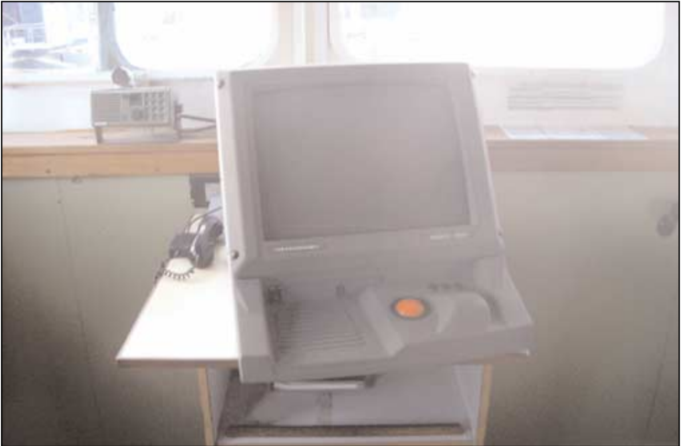
Radar on Briarthorn
