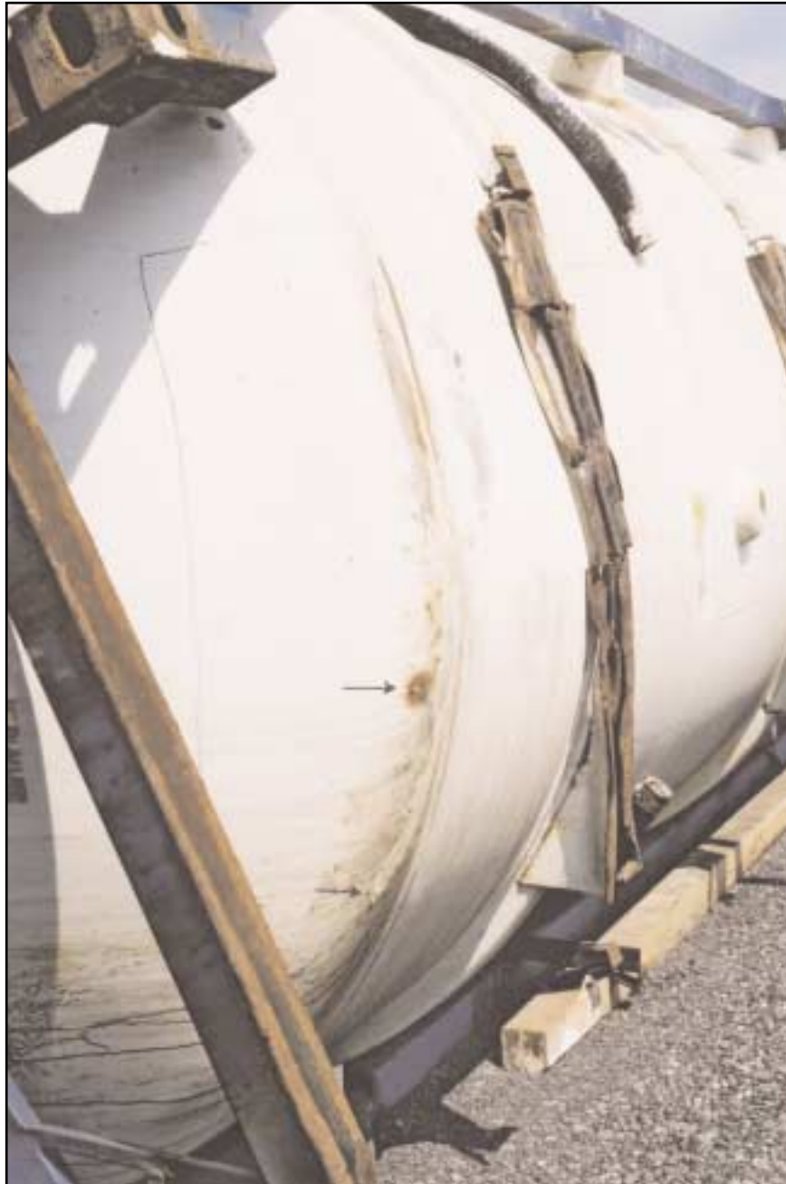
Suspected second leak site and corrosion damage - both arrowed
