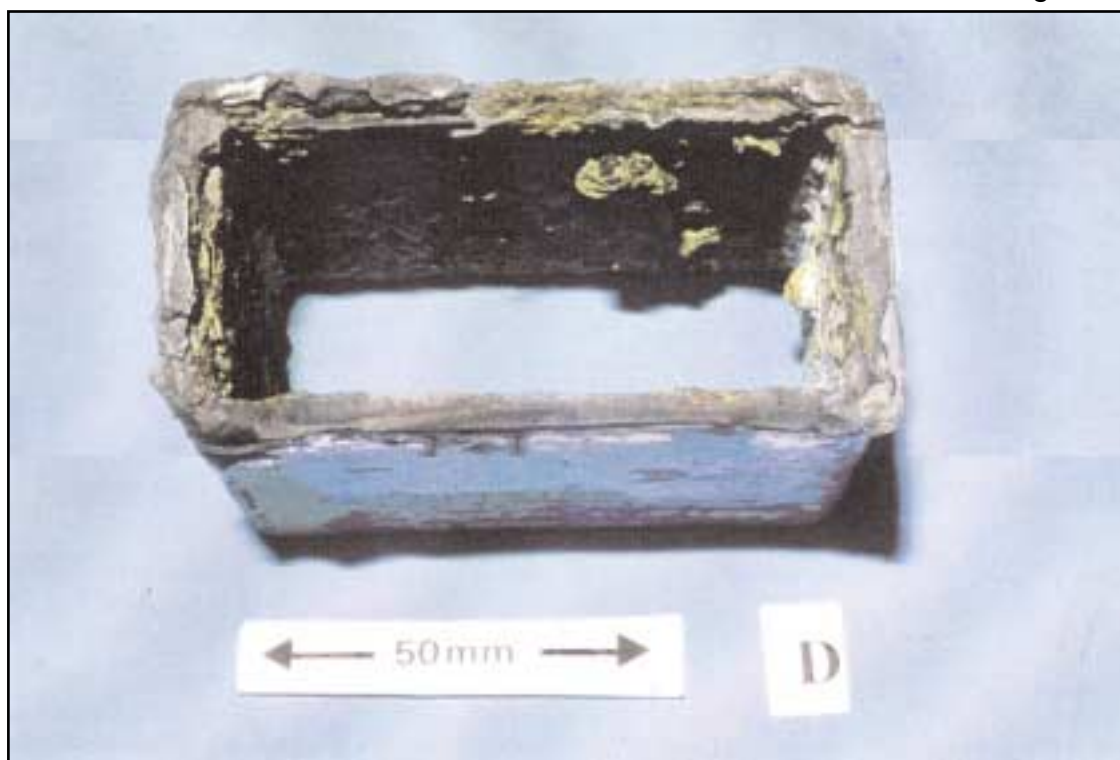
Failed weld repair on rear diagonal
