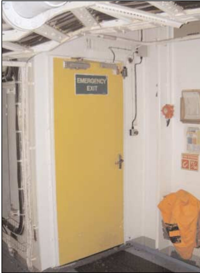
The escape door from No 2 pump room
