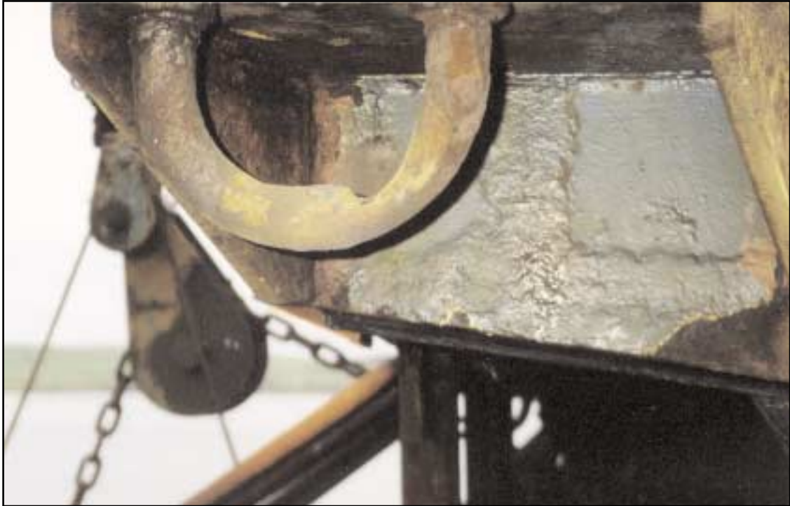
The hanger bolt for the starboard main warp block in-situ onboard Ocean Star
