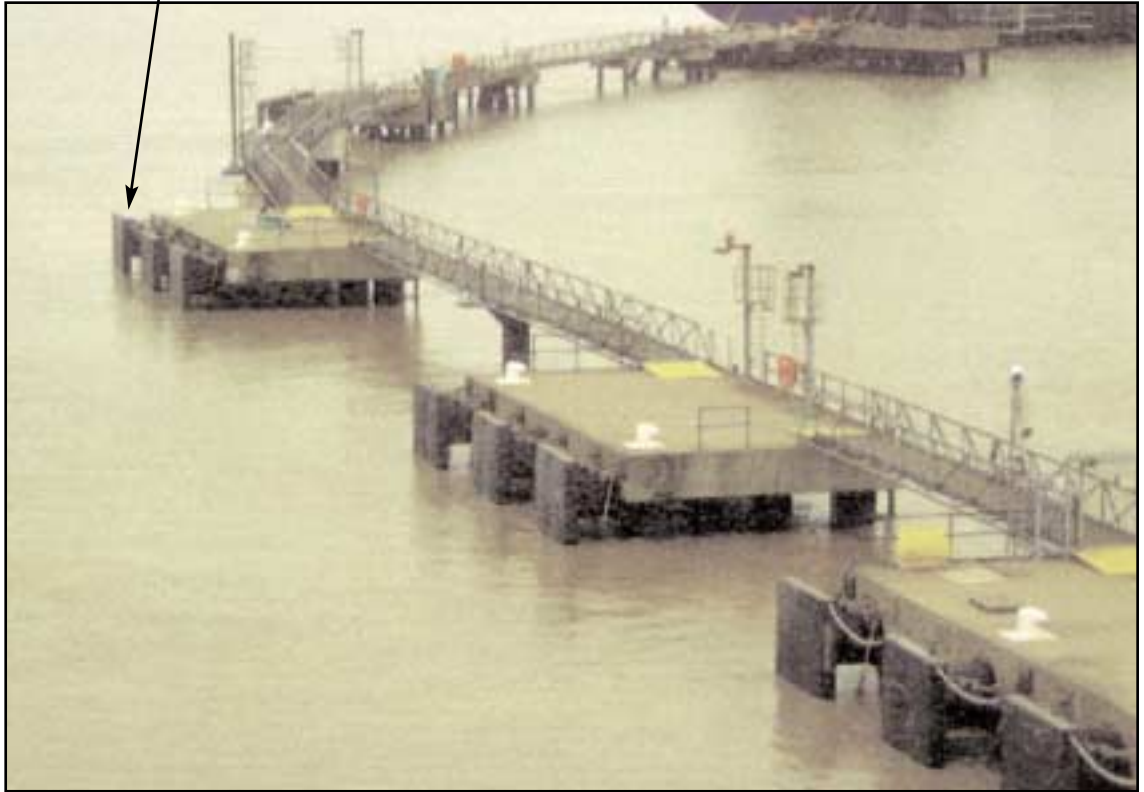
Eastern approach jetty (taken June 2002 after fender repaired)
