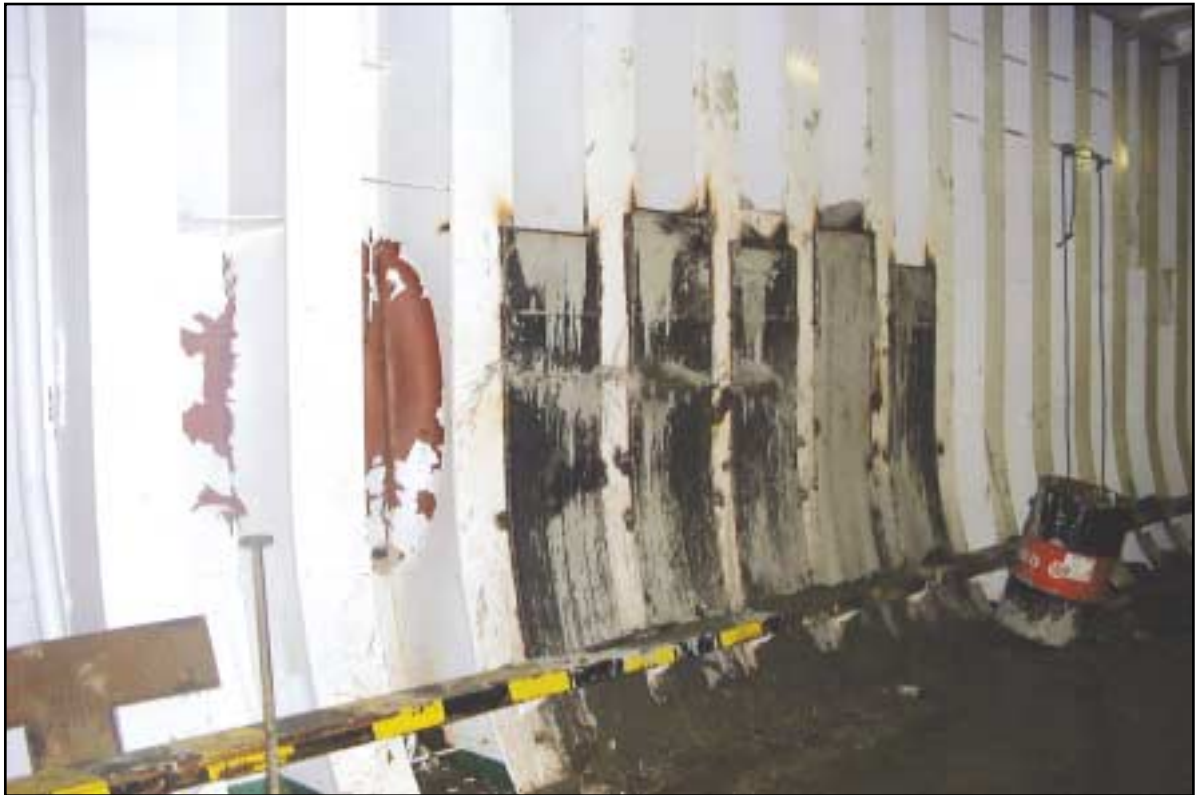
Temporary repair made to damage
