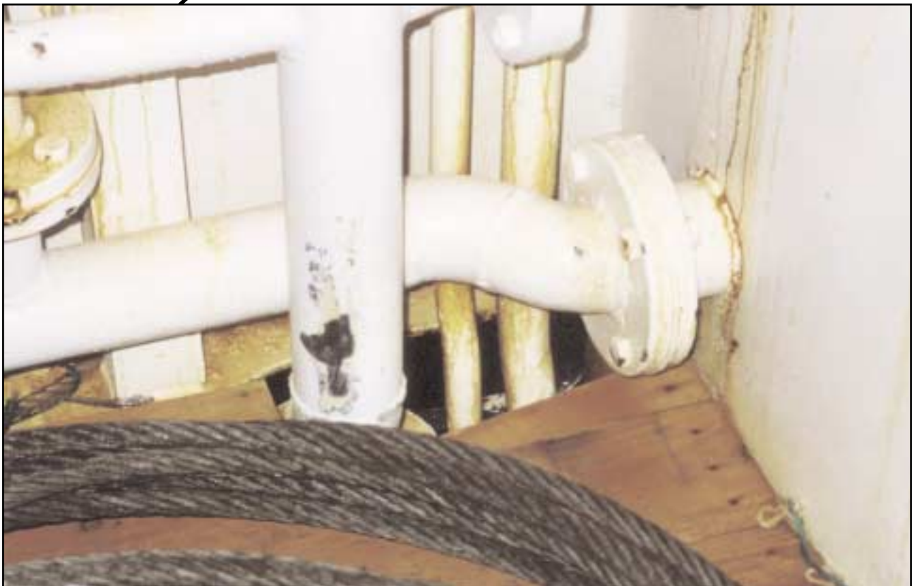
Scupper adjacent to engine air intakes
