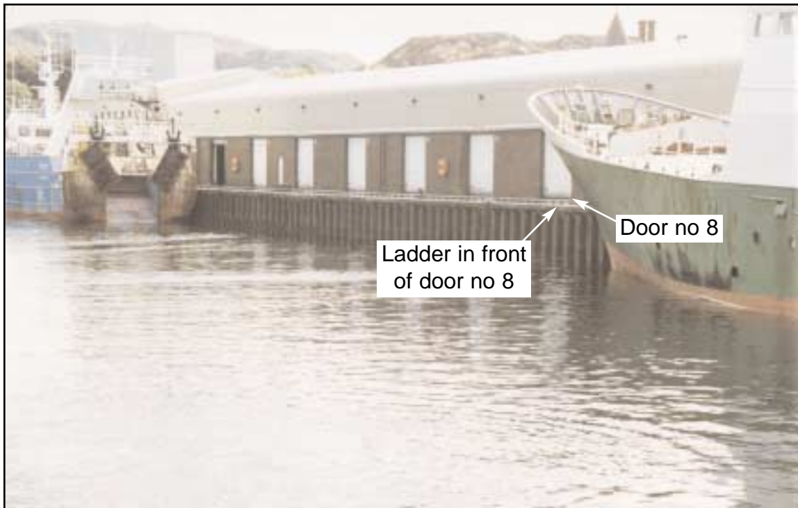
Lochinvar Market Quay (ladder highlighted)
