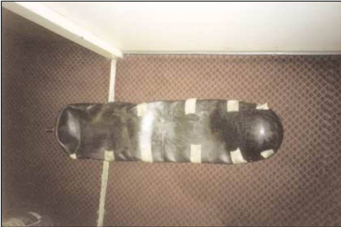
Bladder used to stem flooding (compressed air connection at left hand end)
