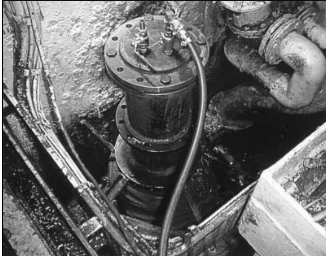
'Top hat' device to insert bellows into leaking pipe
