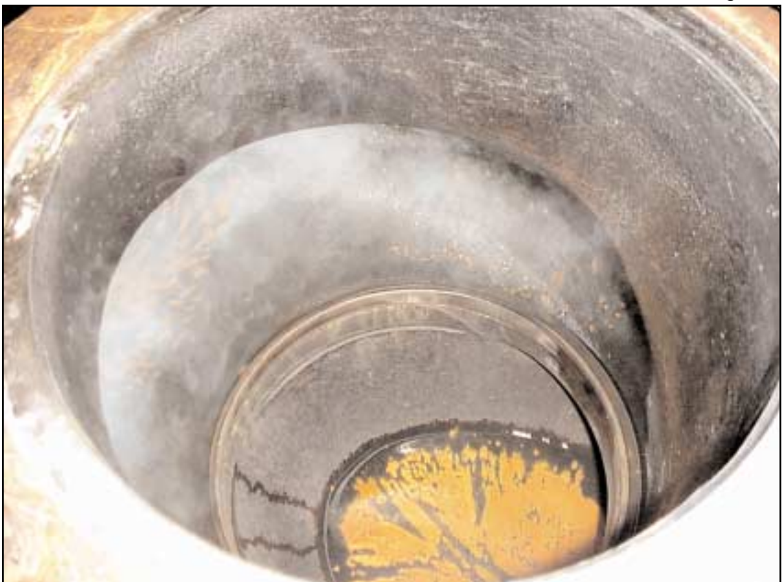
Photograph of valve taken by ships staff
