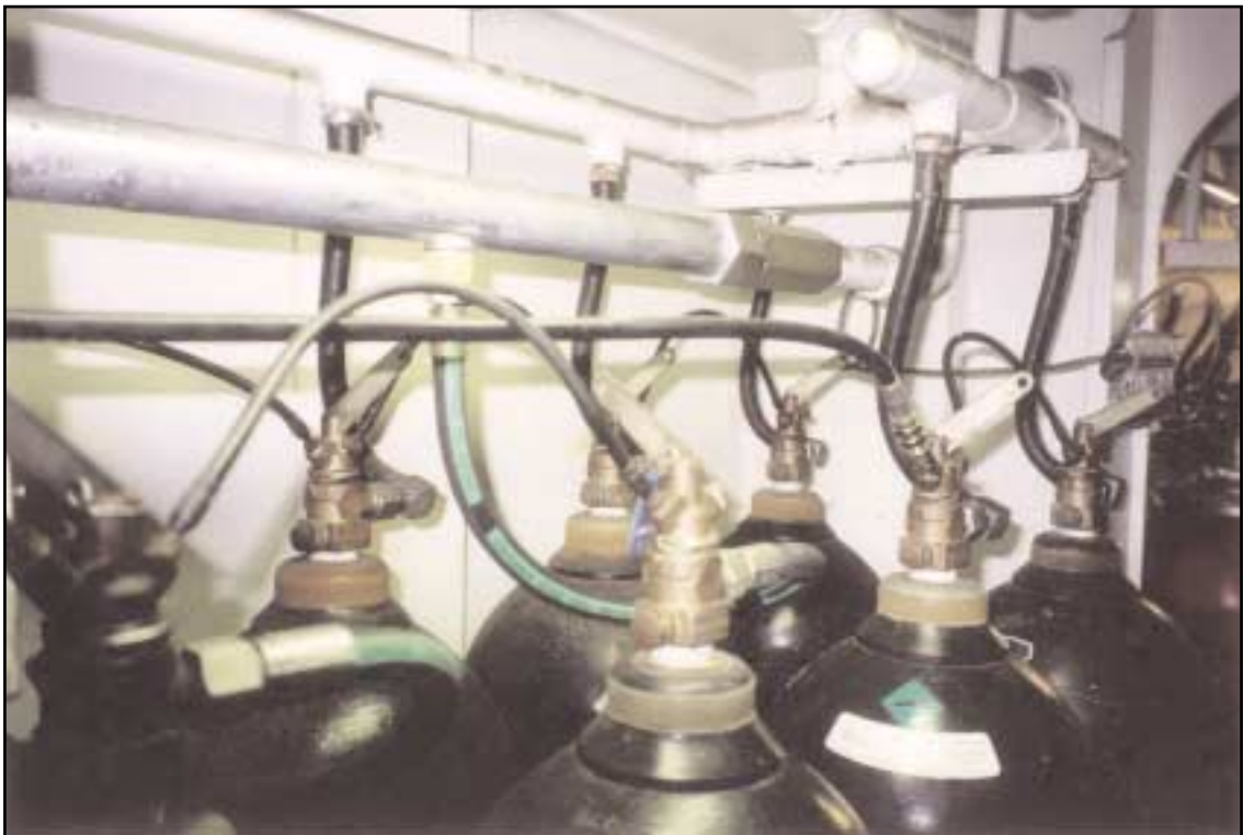
High pressure cylinders in the CO 2 room
