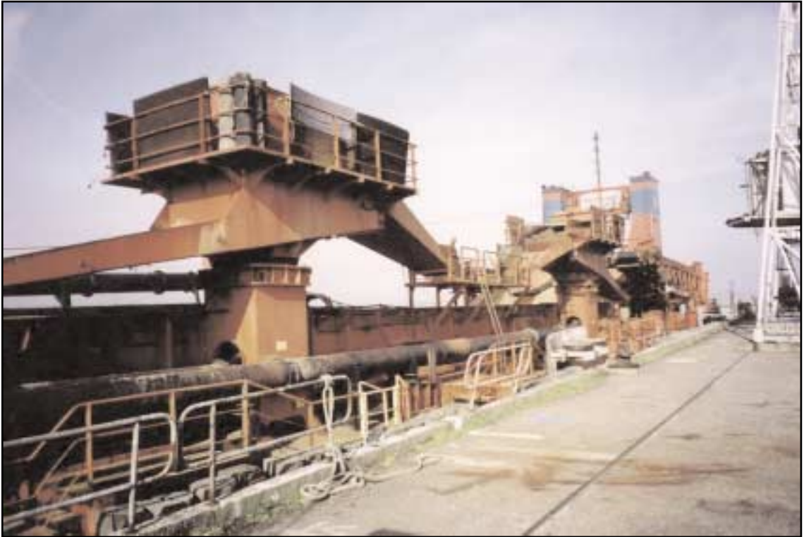
View of loading towers in stowed position
