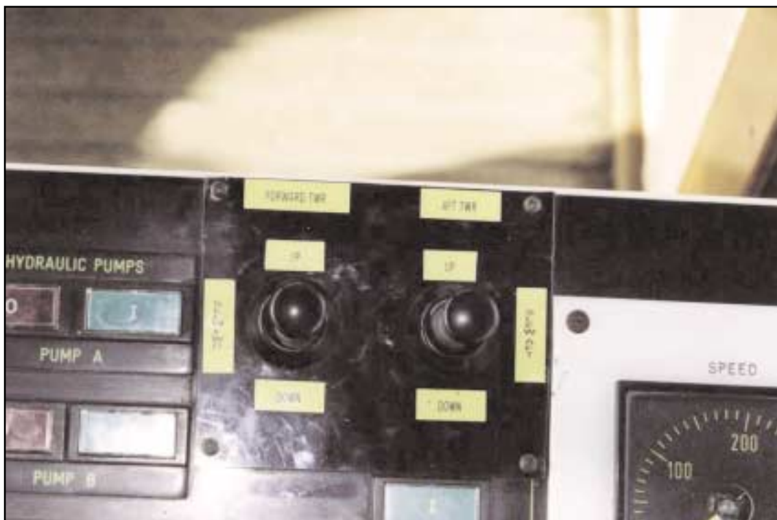
View of loading tower controls
