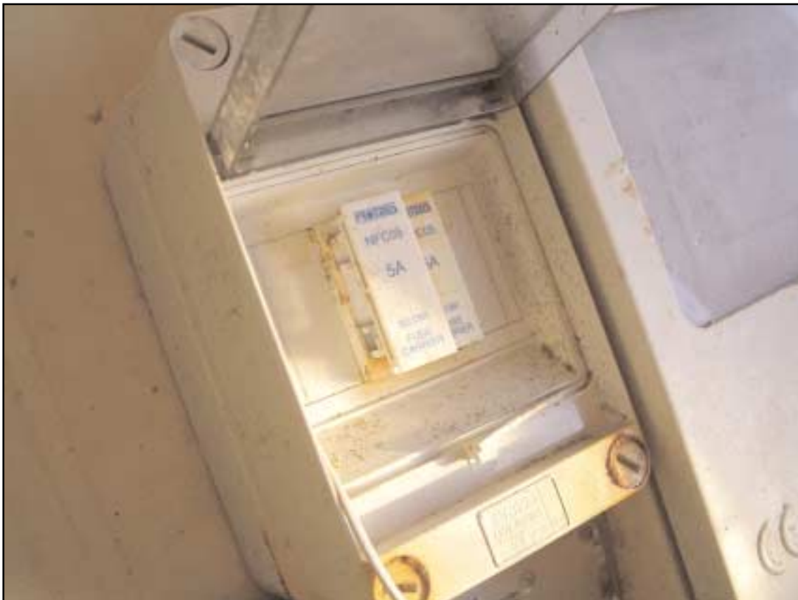
Fuse panel supplying bilge and fire alarms
