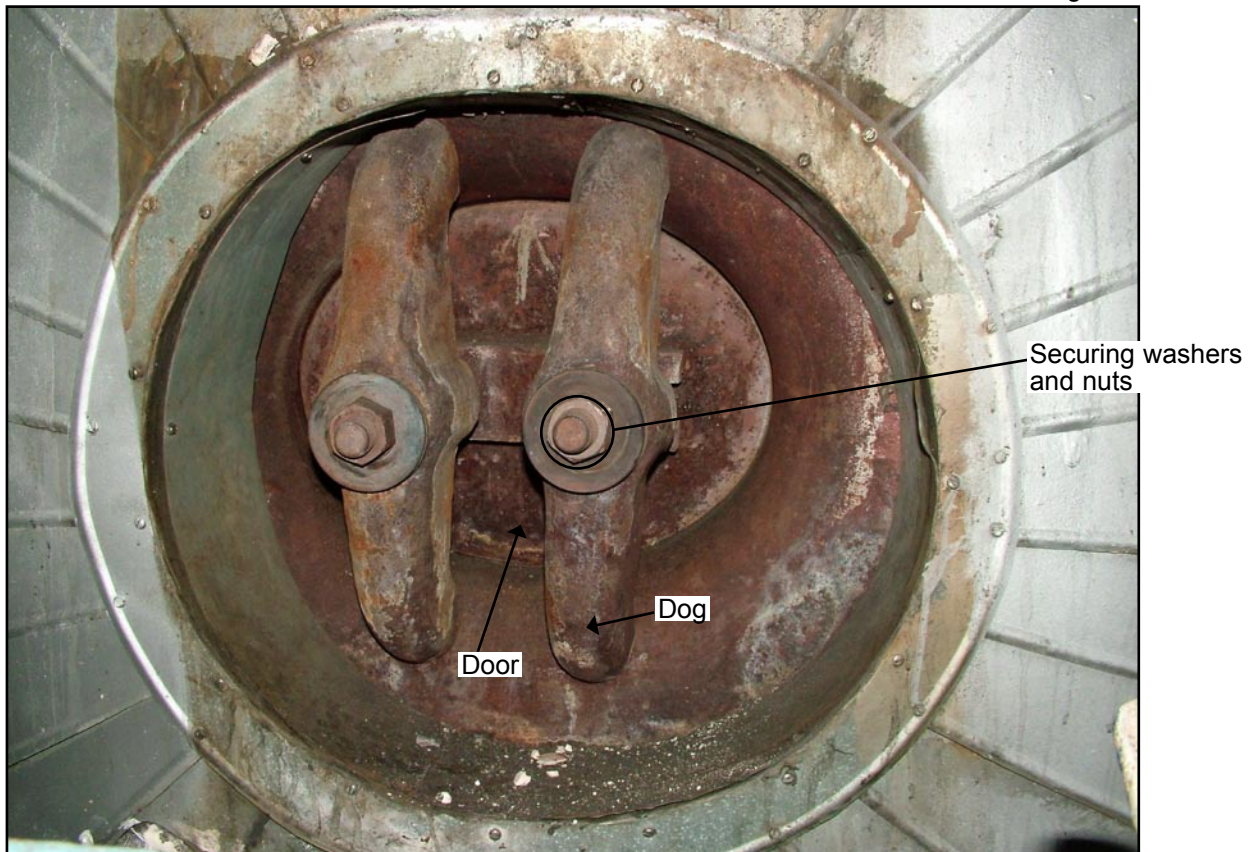
Starboard boiler steam drum, door arrangement
