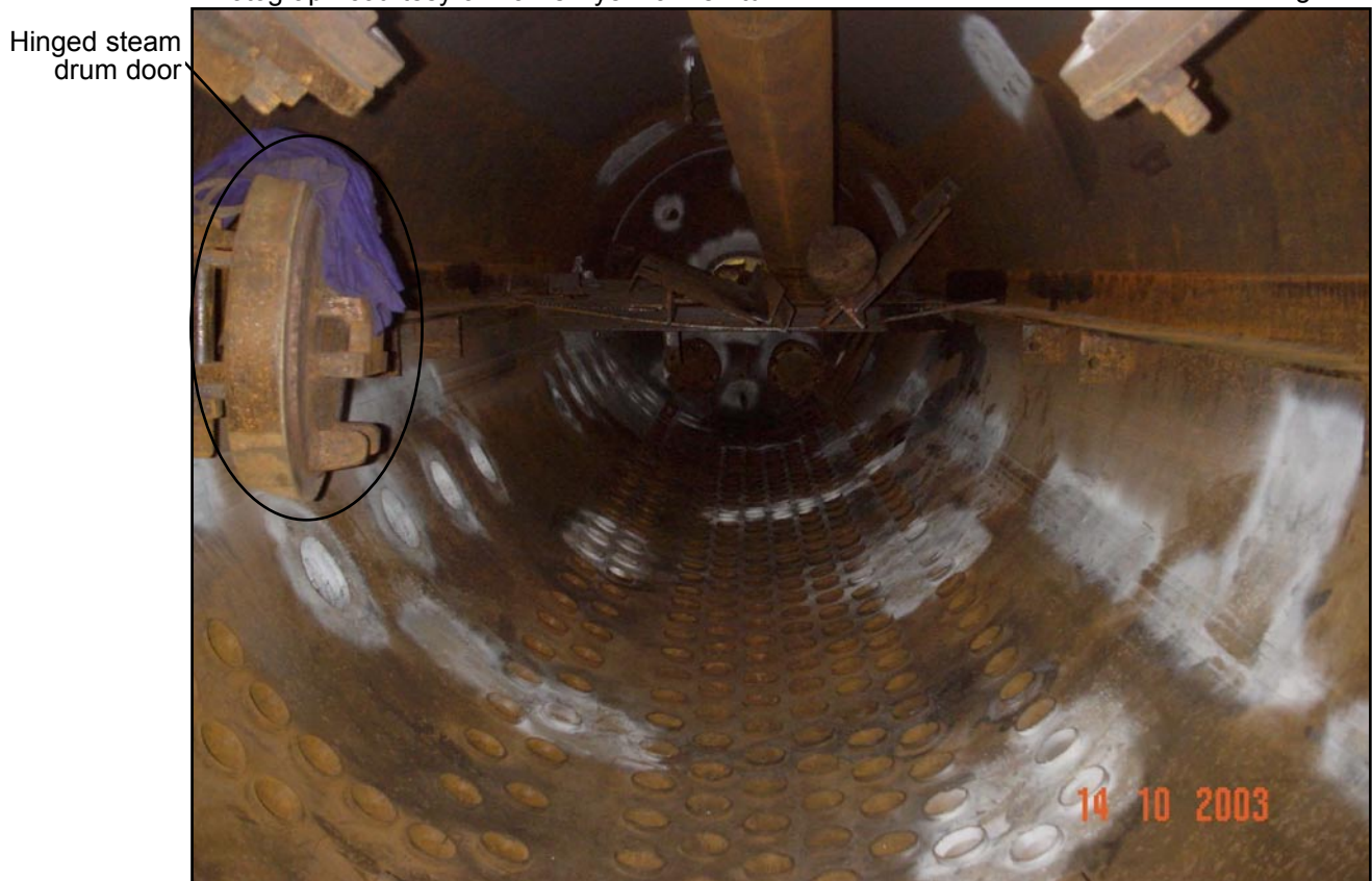
Starboard boiler – open steam drum
