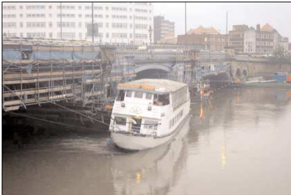
Vessel fast to bridge on Saturday pm
