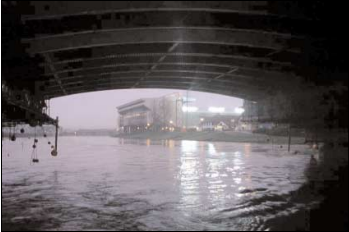
Water flow under centre arch looking downriver
