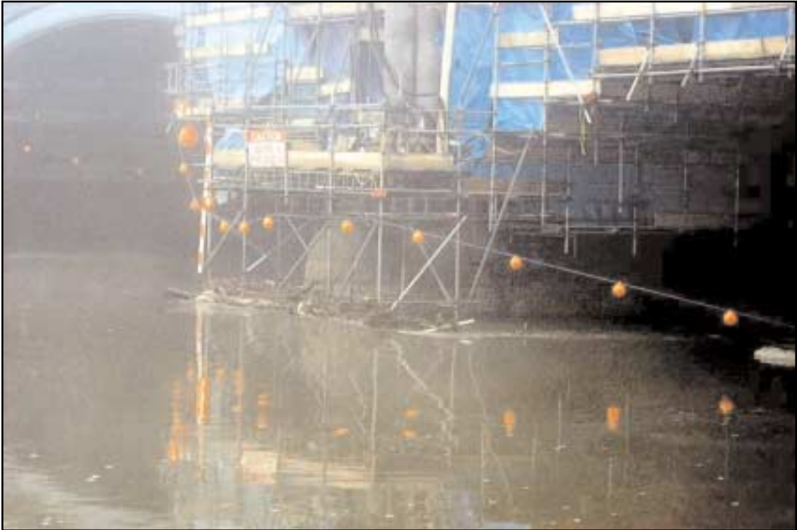
Scaffolding around southern buttness
