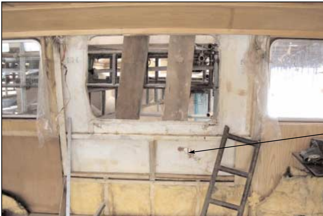
Damage to window on lower deck
