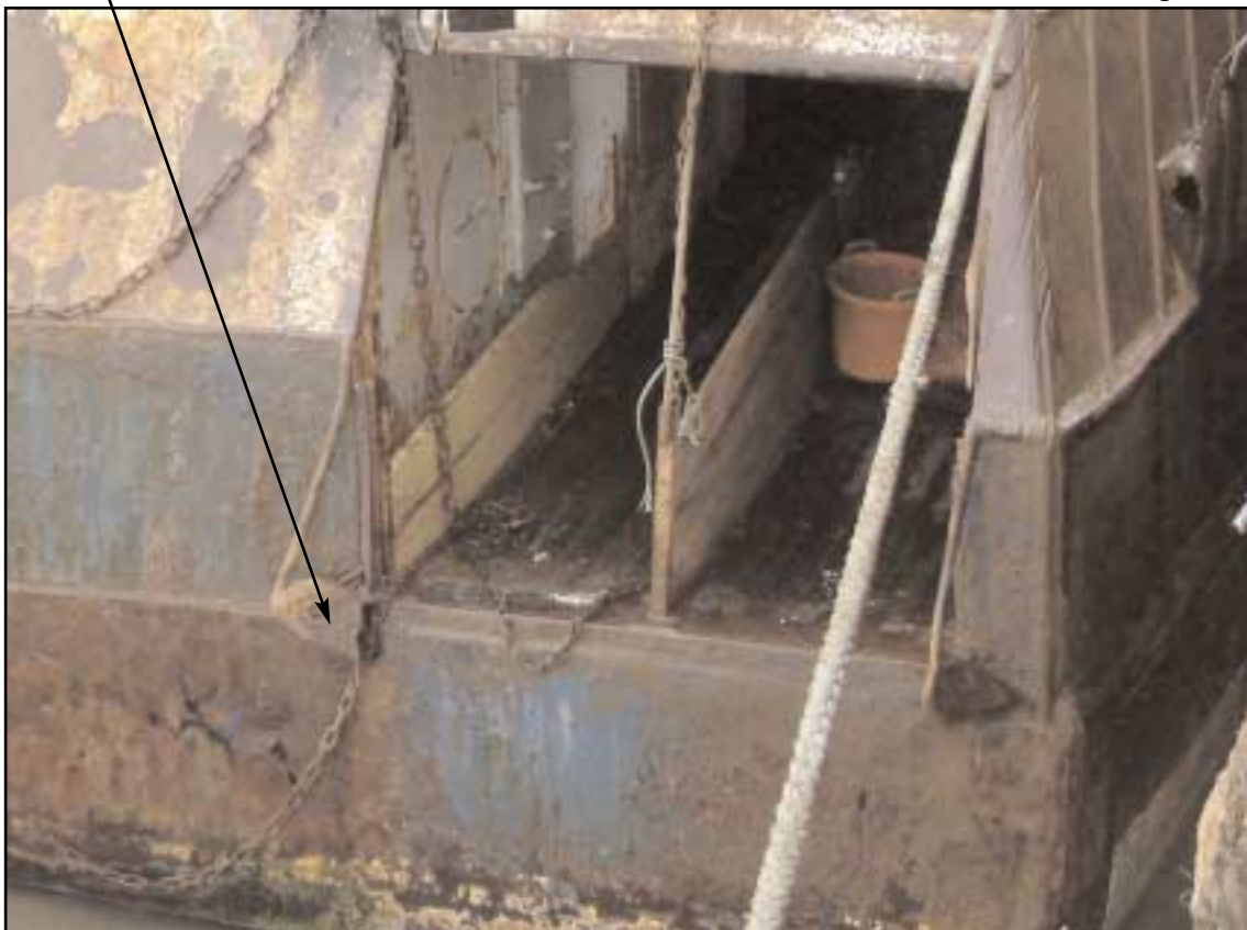
Photograph showing roller fairlead bracket damage
