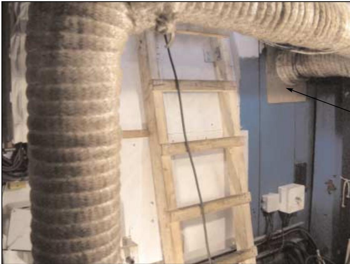
Area of bulkhead penetration. (Now shown with a post repair closure plate.)
