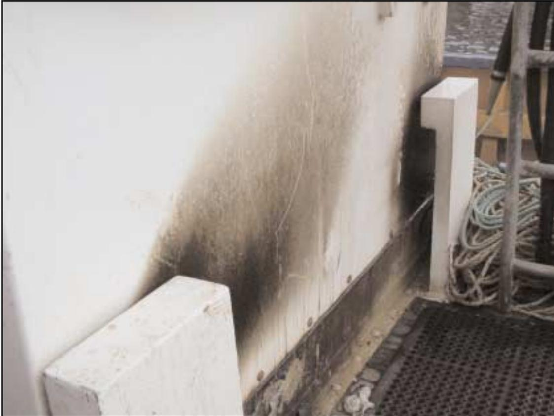
Smoke discharge marks from engine room vents
